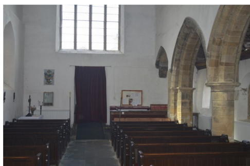
West end prior to works
