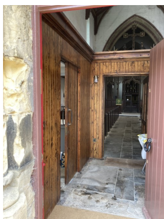
New level access into the church
