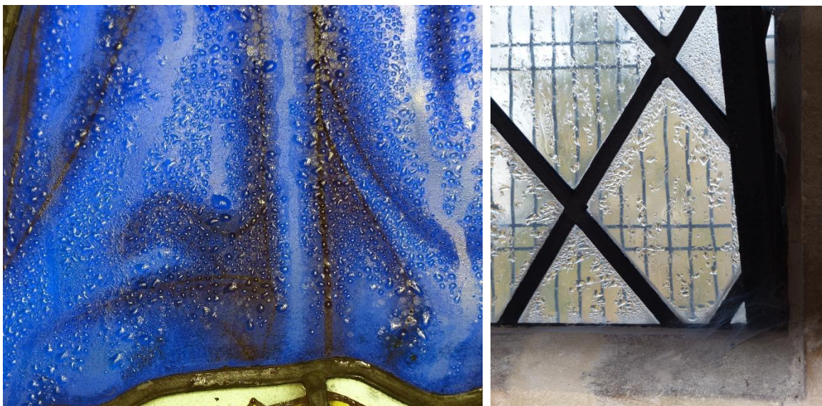
Severe condensation can form on cold surfaces, such as glass, causing damage to adjacent stonework.
