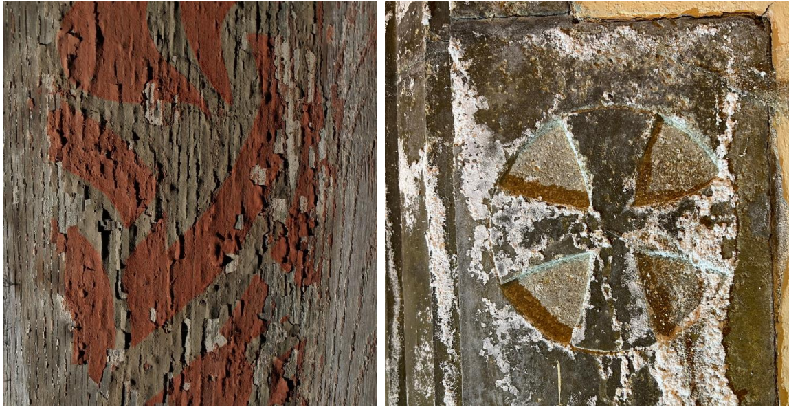
Damage to a painted ceiling and salt deterioration on masonry due to unstable environmental conditions.
