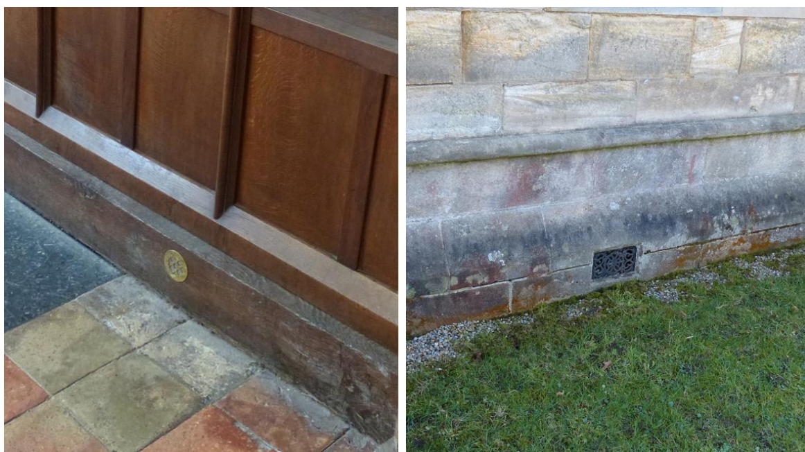
External and internal ventilation openings to under pew voids are designed to reduce moisture levels.
