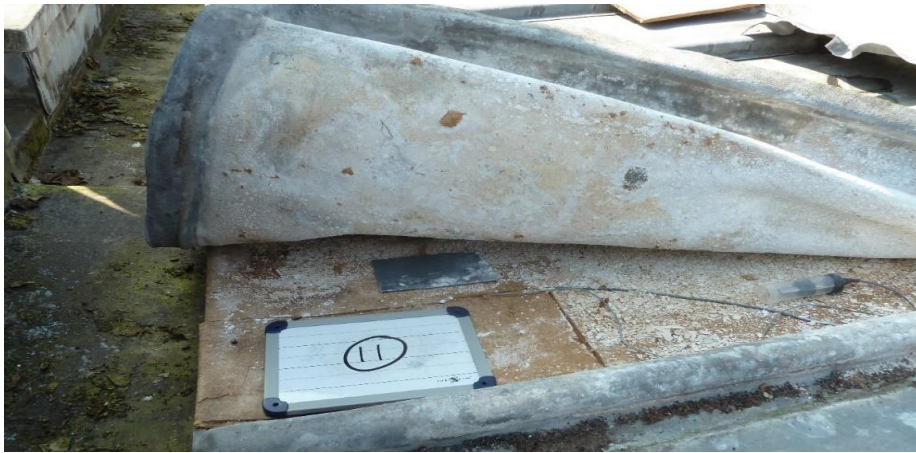
An example of underside lead corrosion: poorly designed roofs with insufficient roof space airflow can lead to severe condensation, resulting in underside lead corrosion.
