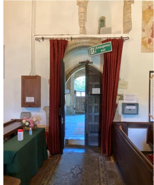
Tower curtains and external door curtains can significantly reduce air movement and draughts.
