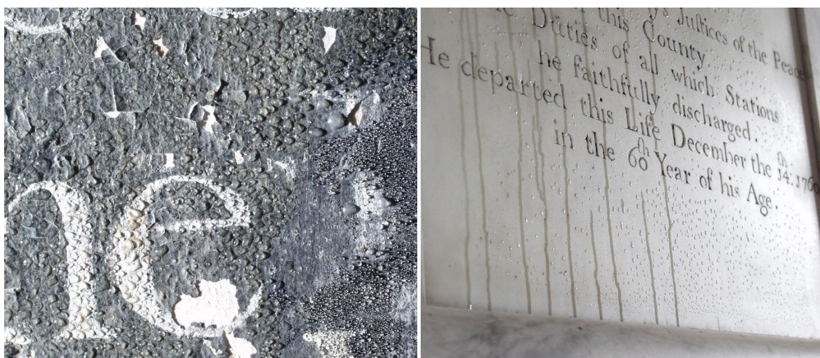
The introduction of warm, moist “fresh” air into a cold church can cause significant condensation and damage.
