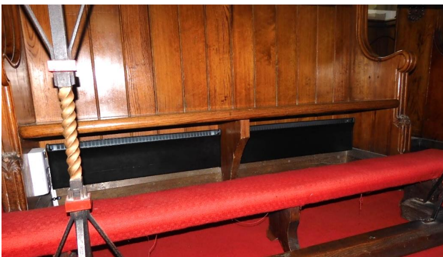
Black 650W Norel under pew heaters fitted to solid pew backs
