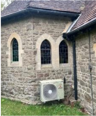
Air source heat pump external unit
