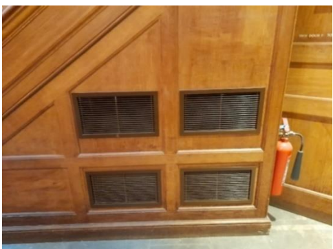
Internal unit installed behind timber panelling at St Andrews in the Wardrobe, City of London – Photo Credits: P Hamley, WCS Services
