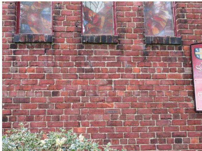
18. The E gable brickwork is good but bellied out from vertical at sill level where some joints are cracked in and below the brick-on-edge sills and two cracked bricks below the sills. No visible change. A cherry tree by the boundary wall is about the recommended minimum 6m away so in severe drought might also influence the wall's foundation. Two other trees formerly near the gable have been removed.
