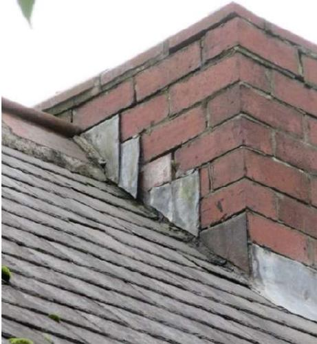
Lead cover flashing missing from NW of chimney
