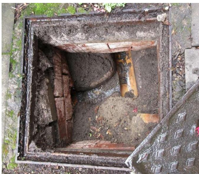
Loose brickwork and soil blocking kitchen branch at NW manhole
