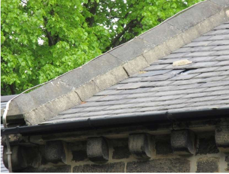
Nave SW corner – hole in slates
