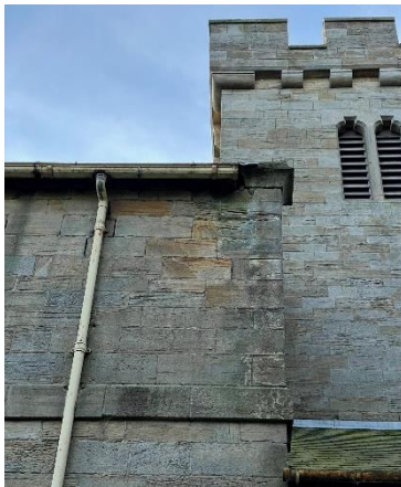
Figure 5- Gutter to north Nave
