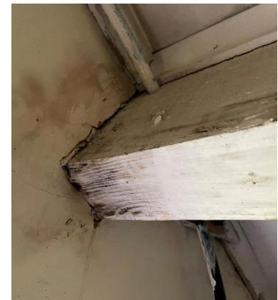
Figure 15- Purlin to upper NW room
