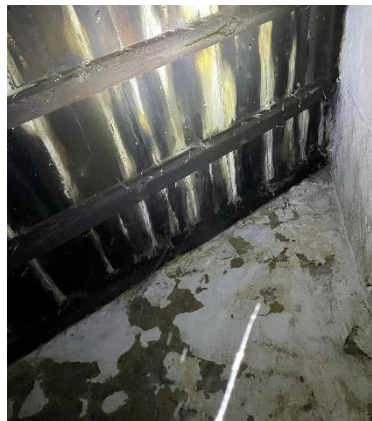
Figure 13- Roof over catslide
