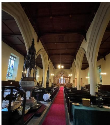
Internal View of Nave
