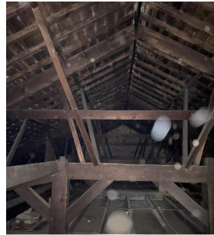
Figure 12 – internal view of Nave
