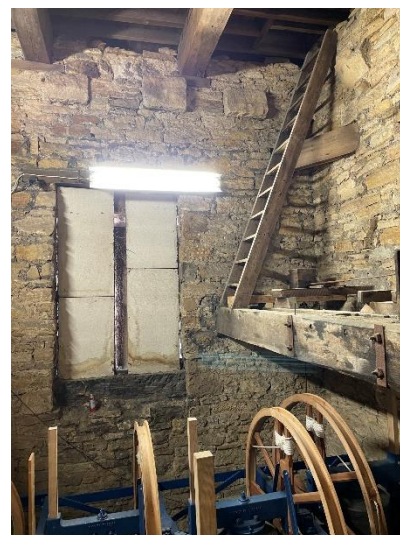
Figure 9- Bells and upper access ladder
