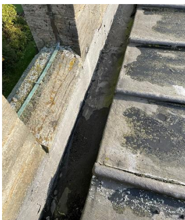
Figure 3- Box Gutter
