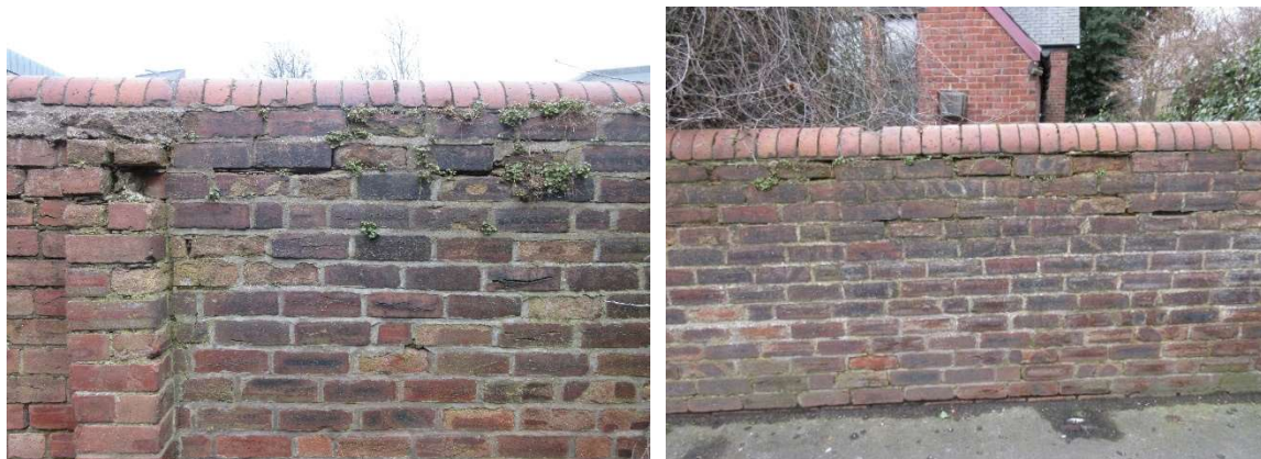
part of the N wall – inside and outside
