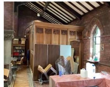
3.55 Flooring generally appears to be in good condition. There are boards where the pews have been removed in the northern part of the aisle and there is parquet along the aisle itself. There is a little bit of unevenness within the transition between the surfaces.
