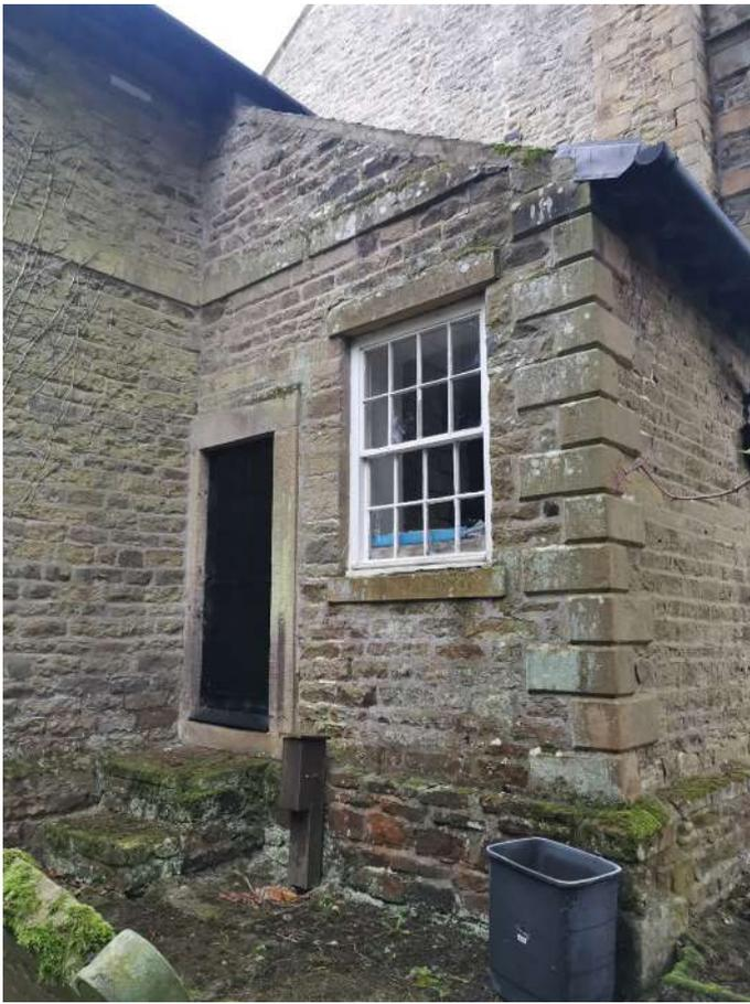
Heavy moss, damp plinth, cementitious pointing - may have caused timber rot to floor internally
