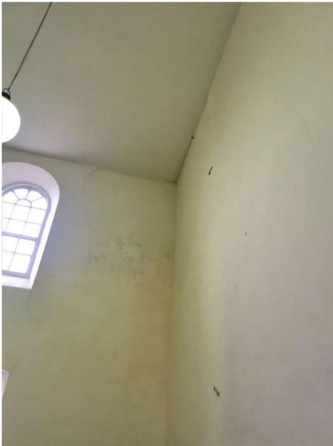
New crack in plaster to west of western window, damp damaged finishes. Tell-tale to western wall
