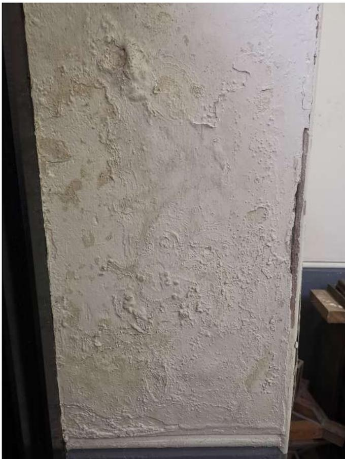
Internal walls of tower worsened - non-breathable paint making issues worse
