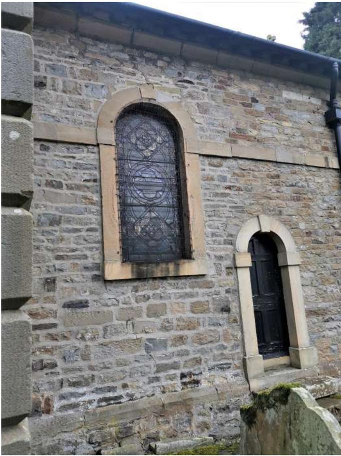
Cracks through masonry and bulge over window
