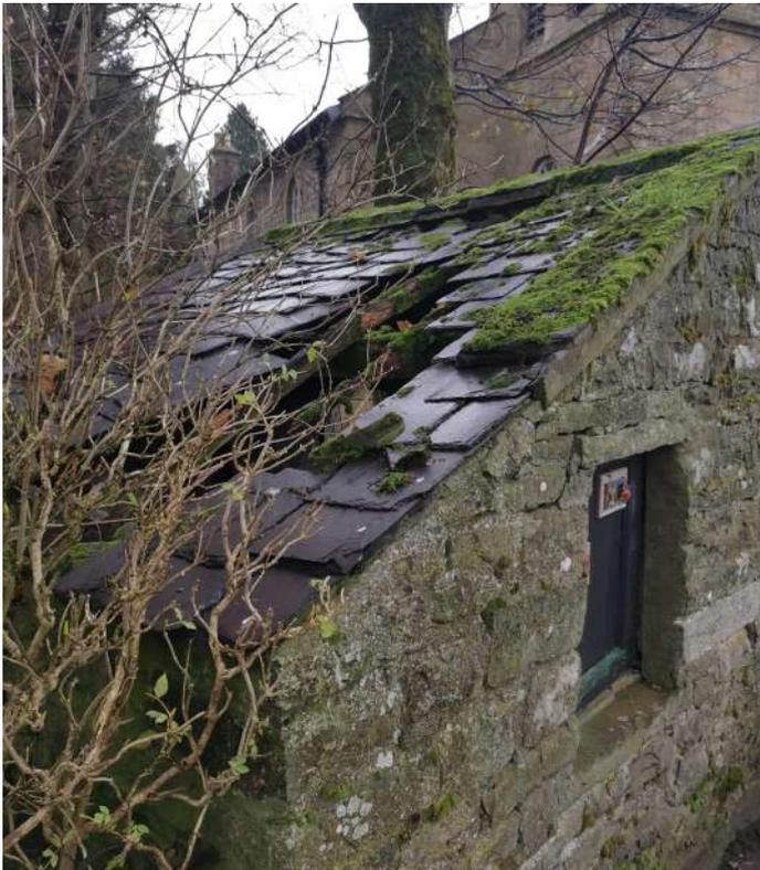
Garden shed roof collapsed - dangerous. Northern wall of shed/boundary wall also collapsed at eastern corner
