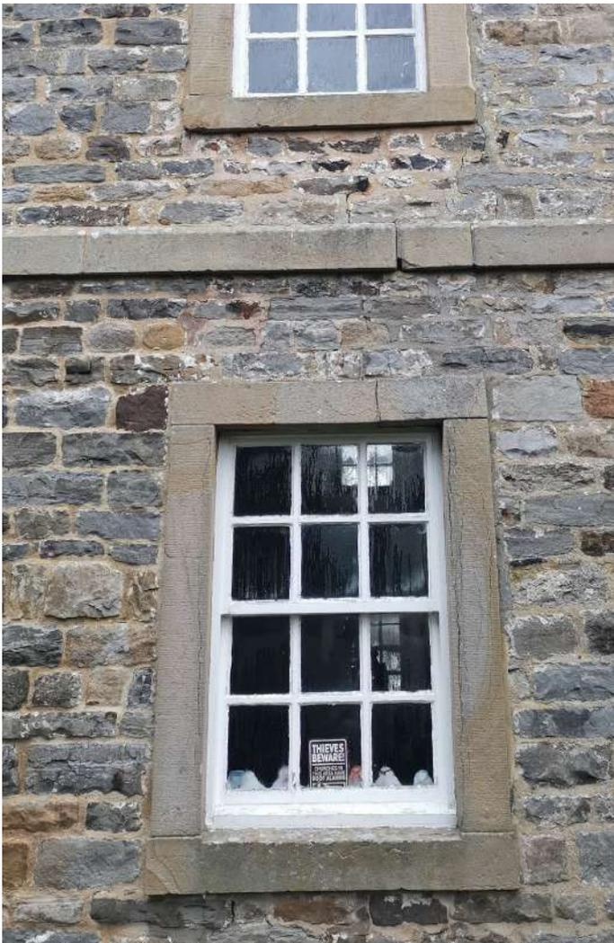
Splits down vertical window jambs. Cracks through head lintel and stringcourse above.
