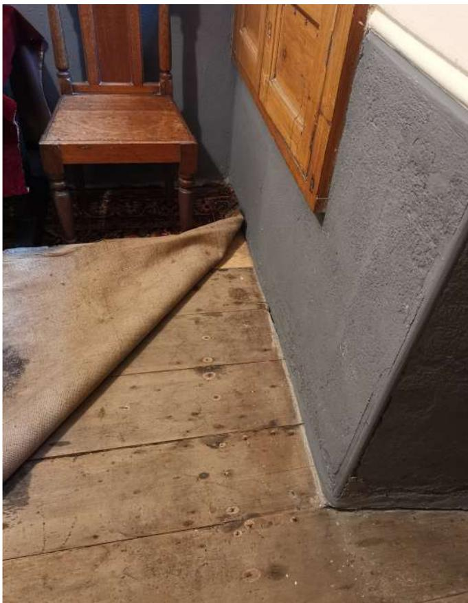
Area of floor to east vestry wall is spongy underfoot indicating lack of support, possibly rotten joists
