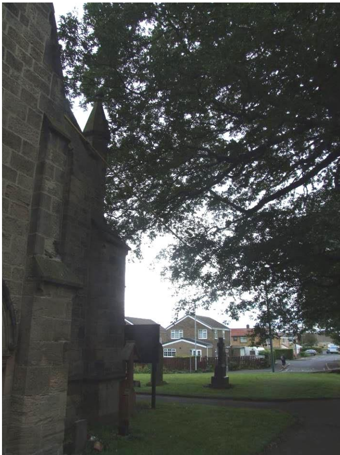
P29 (8868): Tree proximity, west end
