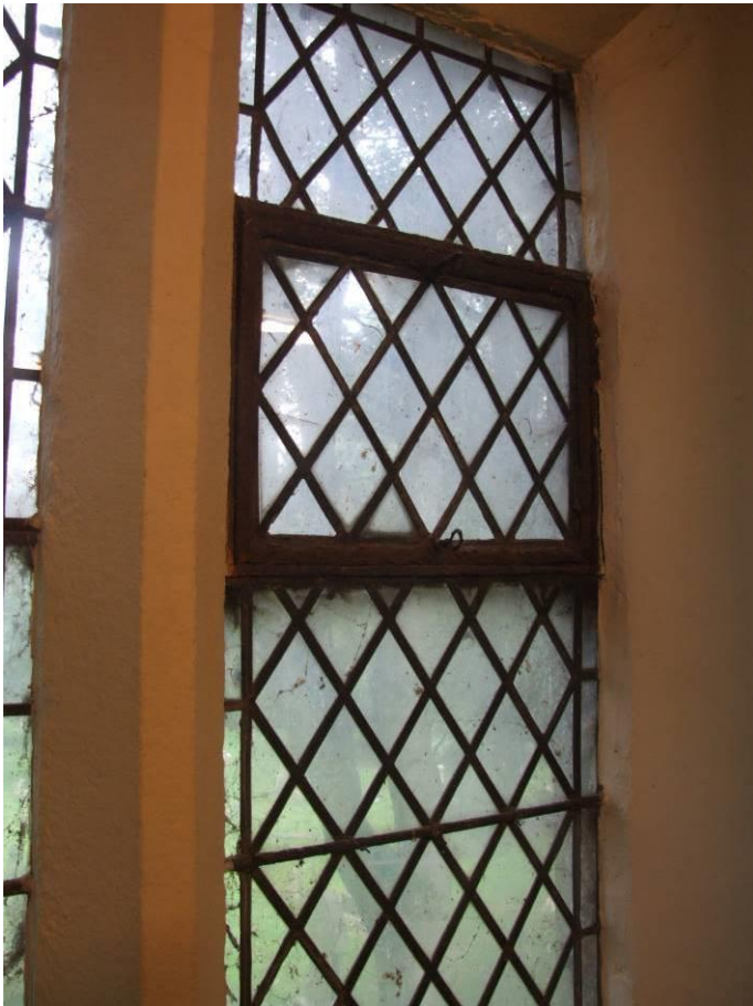
P17 (8850): Vestry opening lights, no longer operable
