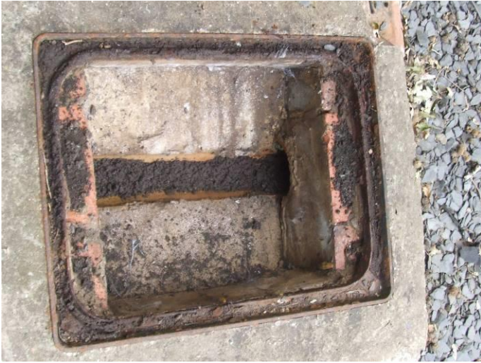
P25 (8860): Surface water manhole, south side nave
