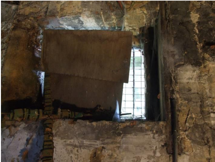
P12 (8829): Boiler room window opening
