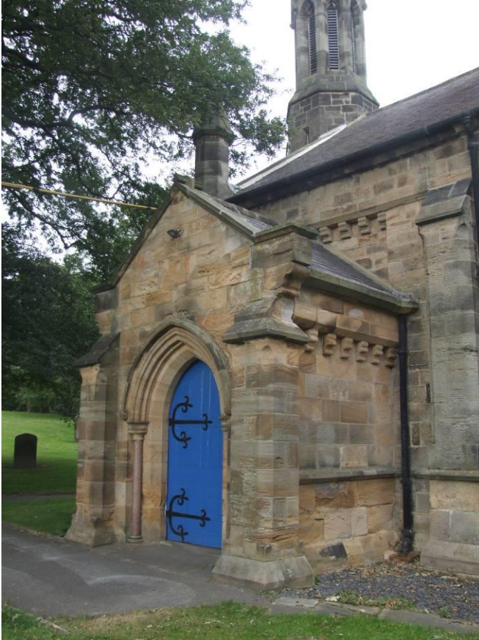
P23 (8858): South porch, extension
