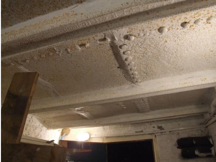
P11 (8826): Store room ceiling; second-hand boiler plates and rail structure
