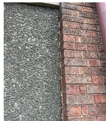
Figure 12 – Gap in aggregate panel
