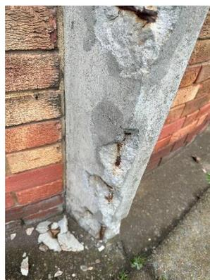
Figure 10 – new spalling
