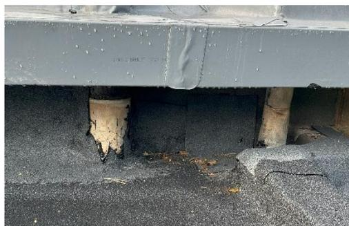
Figure 5 – Felt finish to pipe penetrations.
