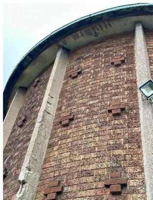
*Figure 34 –Apse Concrete fins*
