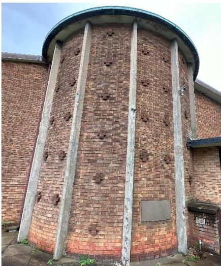
Figure 7 – Apse concrete fins
