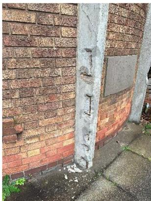
*Figure 35 – Reinforcement exposed*
