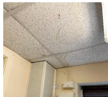
Figure 26 – Staining to kitchen ceiling
