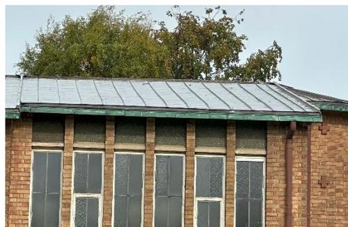
Figure 1 - Undulation to copper roof and debris on top
