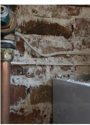
Significant efflorescence to brick joints
