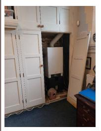
Door to boiler cupboard not fixed. Presume removed to allow access to boiler for maintenance and/or to allow space to dry out see below Re-hang cupboard door.
