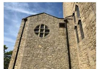
4. South Transept round window W13 has Thompson & Snee stained glass in poor condition with several serious cracks: unprotected.
