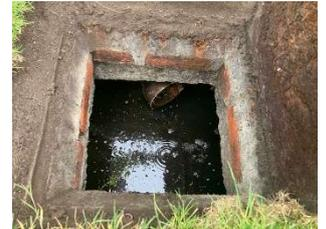
3. Clay dishtops replaced to south and east (2019). Several have deposits of leaf debris.
