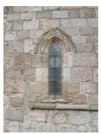
The chancel wall has a general outward bulge in the centre area together with some vertical settlement cracks and open perpends, all of which need re-pointing. Previous pointing is regrettable and unsuitable. Two south facing windows have missing hood mouldings. When funds allow, these should be replaced and made to match the adjacent window hood.
