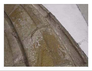
2.2 Of greater concern is the evidence of continuing and accelerating water ingress to the north aisle roof and wall:
