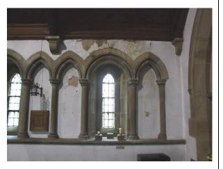
Evidences of water penetration to the north aisle appear to have accelerated over the quinquennial period, during which a Listed Places of Worship Roof Repair Fund bid was unsuccessful).
