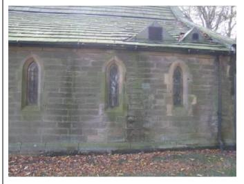
4.2 The downpipes require regular repainting and uncaulked joints in both downpipes and gutters can cause moisture saturation of wall foot and wall head respectively.
