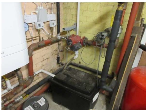
Scope for economy by more lagging at pipes and pump
