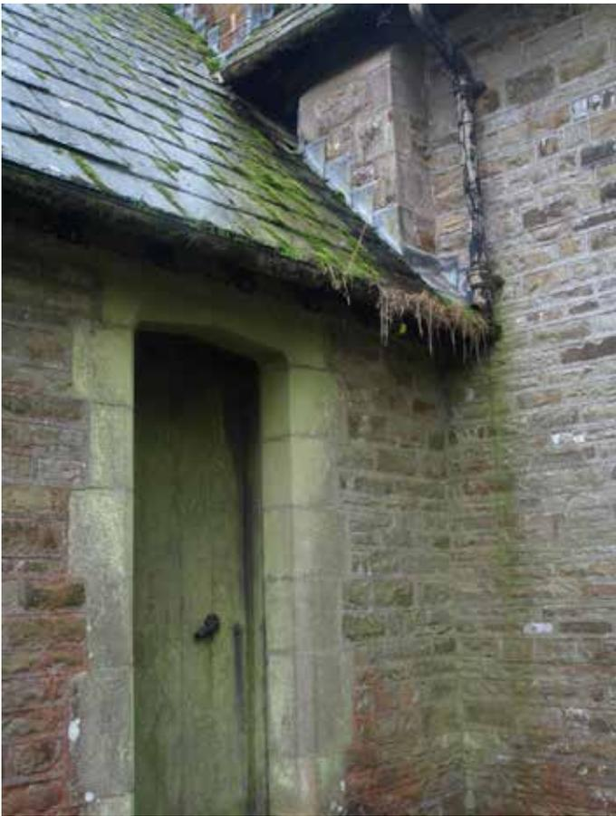
Gutters are full of debris and vegetation in places. Clean out every 6 months to avoid overflow and resultant water ingress
