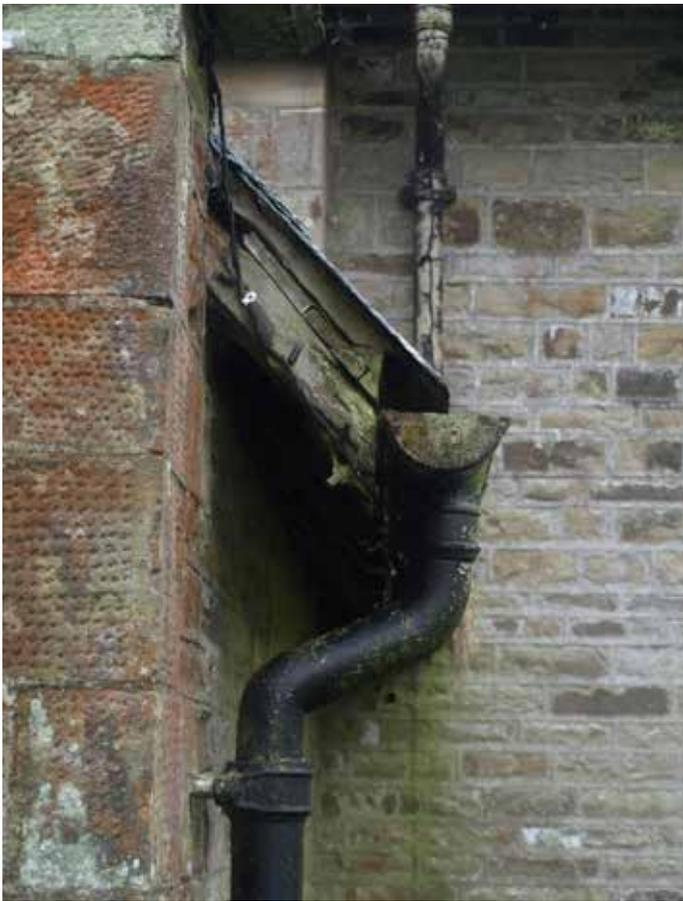
Rafter ends in poor condition, and covering bargeboard missing
