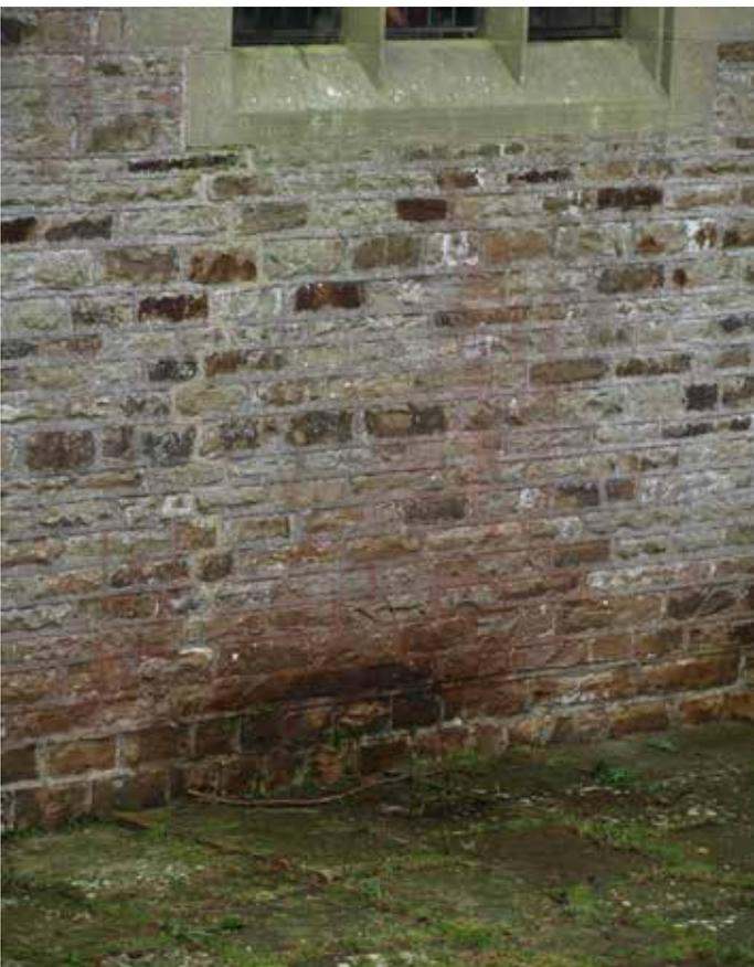
Splashback from leaking gutters causing damp walls
