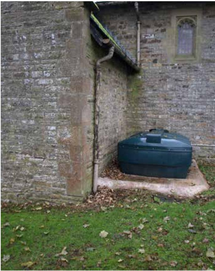
The plinth to the recent oil tank has been built above ground level against the Transept wall, causing damp to the base of the wall internally
