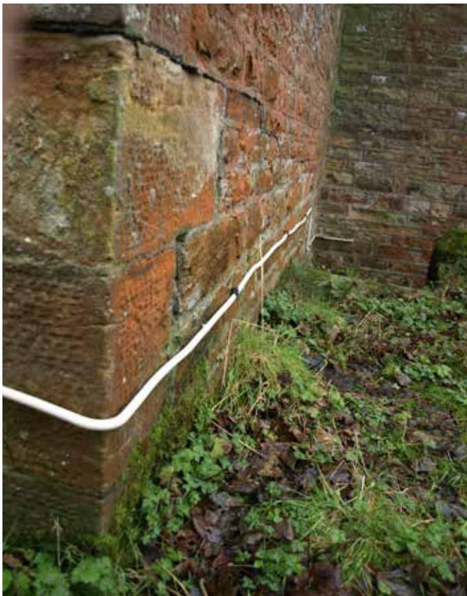
New feed pipe to boiler from recent oil tank installation
