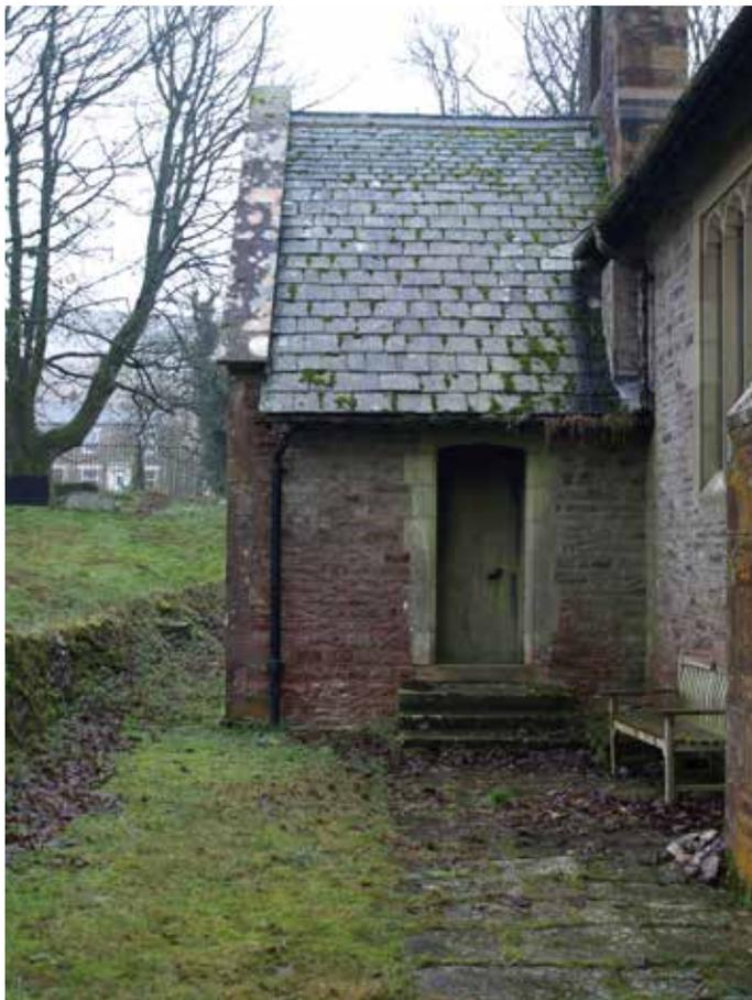
A build-up of vegetation around the building encourages damp conditions and prevents drying of the ground and walls at low level
