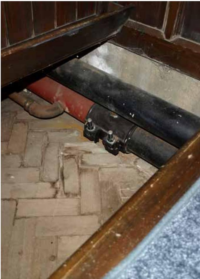
Recent heating pipe repairs have stopped the leaks which were affecting areas of the woodblock flooring
