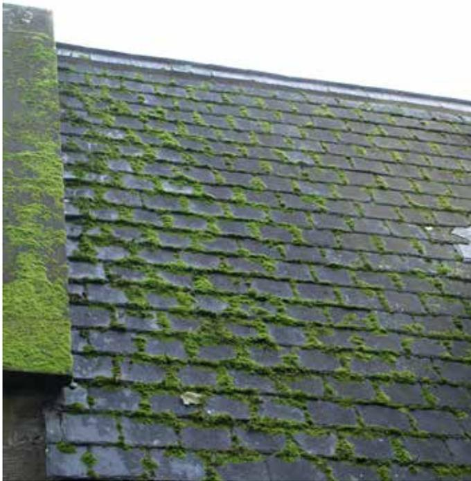
Moss build up encouraged by lack of light and proximity of trees. Will hold water in the slates and prevent ventilation. To be removed
