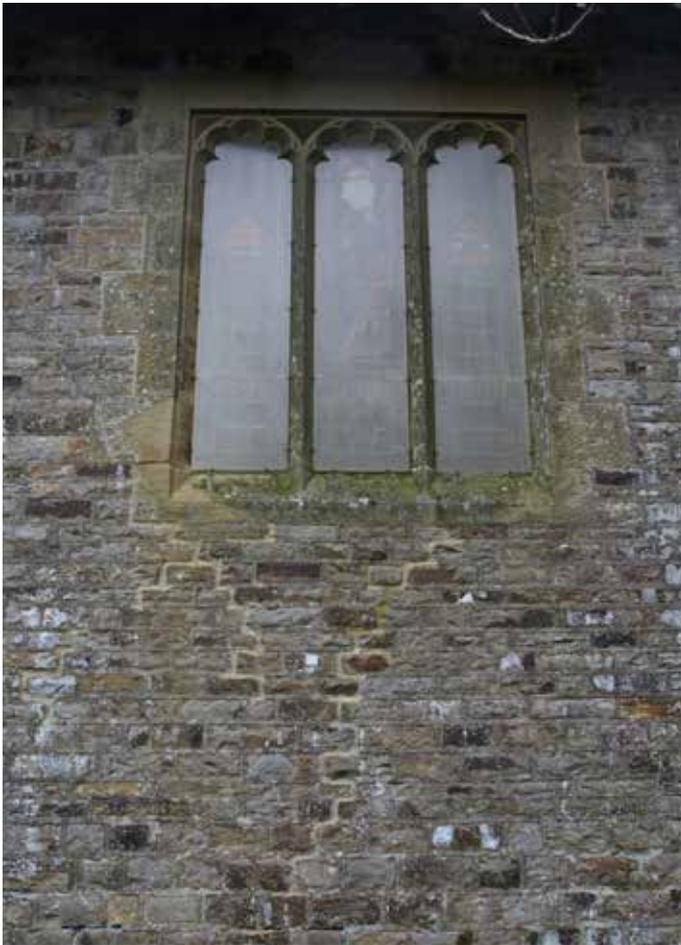
Earlier cracking below south windows, pointed up and in places opening up again
