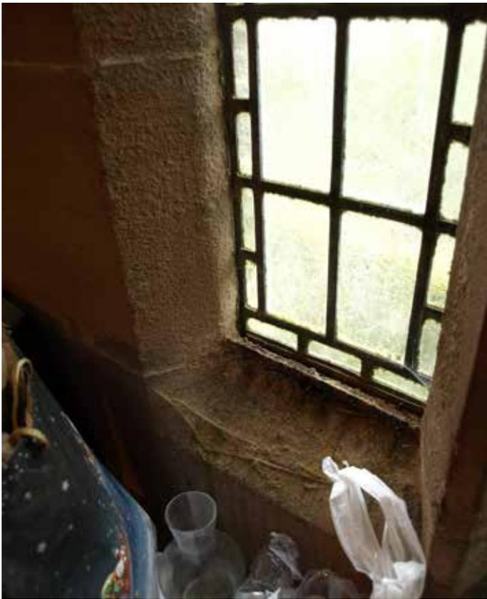
Vestry window (nII) in poor condition due to algae, stone decay, rusting metalwork
