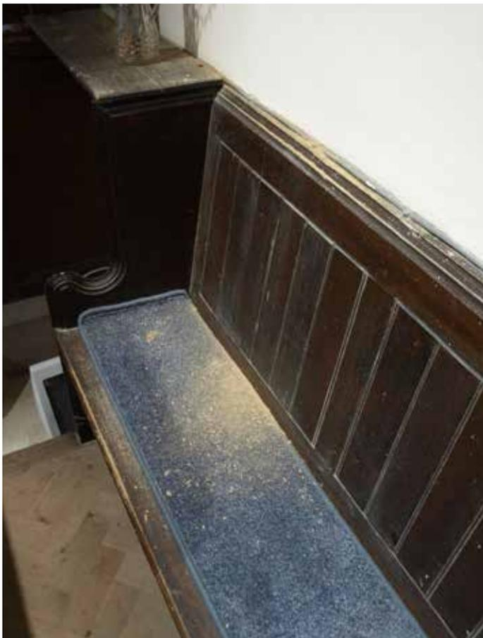
Deposits of stone dust are indicative of the rate of decay. This should be removed by vacuum cleaning
