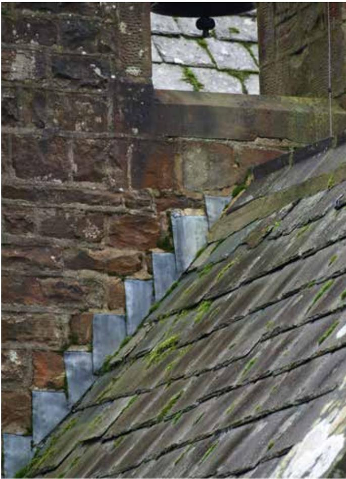
Masonry to the bellcote requires fully re-pointing. Ideally the structure should be re-built on a lead tray
