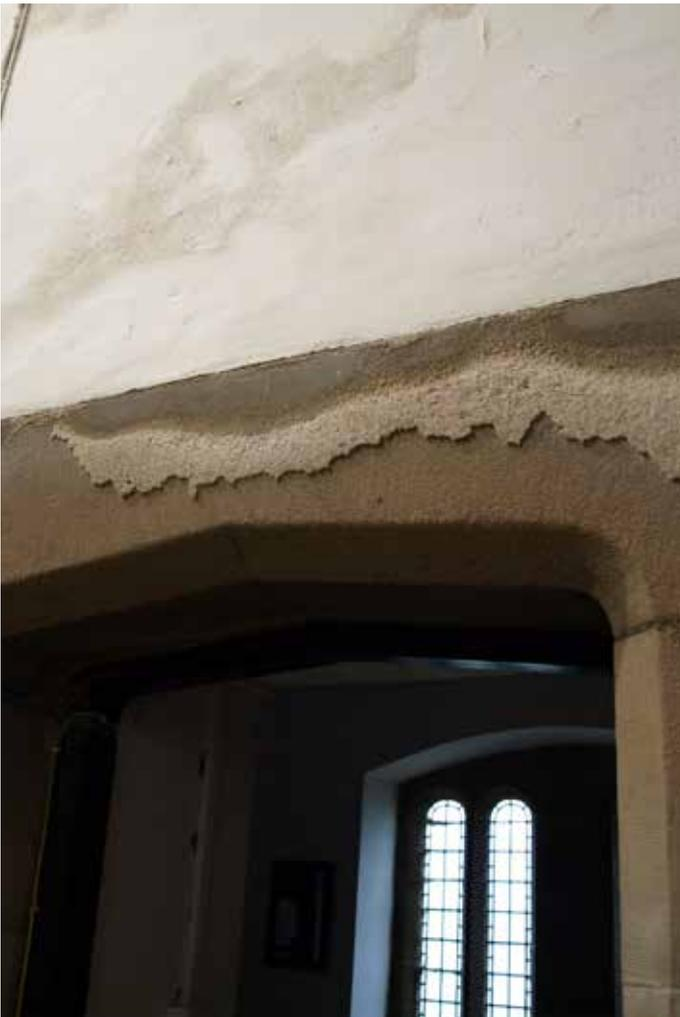
Wall over the Vestry door is wet, causing stone decay to the door surround. Due to leaking bellcote above
