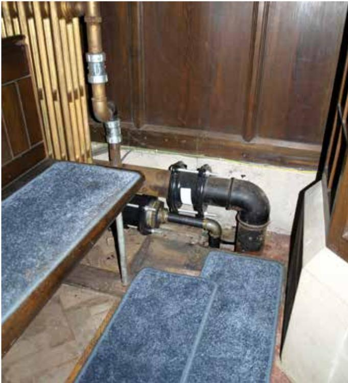
Floor trench to be filled following recent heating pipe repair
