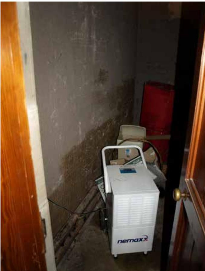
South Transept is extremely damp. Fix sources of ingress, remove plaster from walls, provide drain for dehumidifier so it can work, increase ventilation
