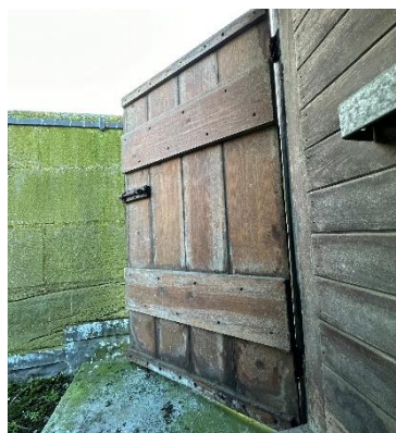
Figure 5 - Tower roof and hatch
