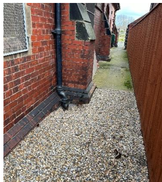
Figure 38 – new fence and gravel
