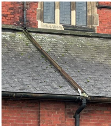
Figure 9 – Channels on N Aisle roof
