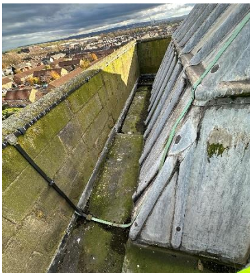
Figure 4 - tower lead gutter
