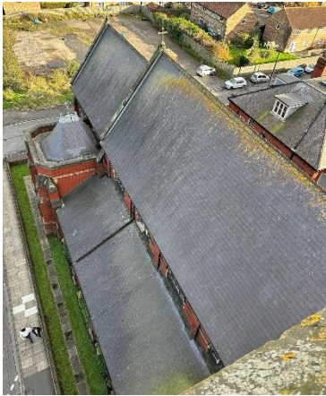
Figure 7- Roof from tower
