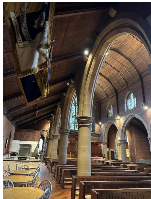
Internal view of Nave
