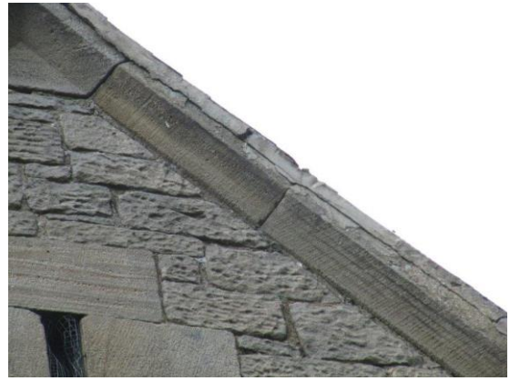
Hungry joints to the Gable of the east Elevation and failing mortar to verge
