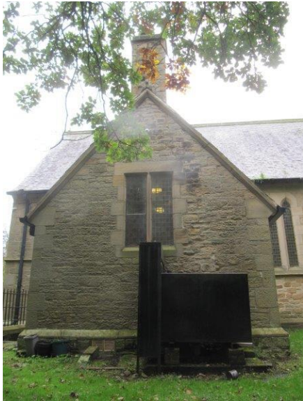
Oil tank location in close proximity to the Vestry
