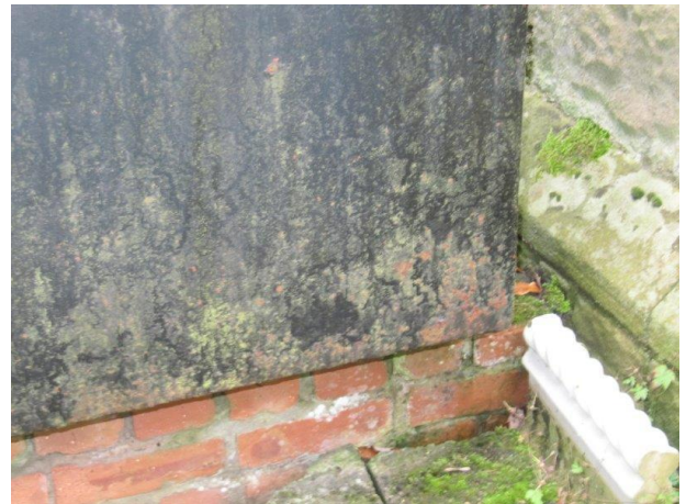
Rusting base to the oil tank
