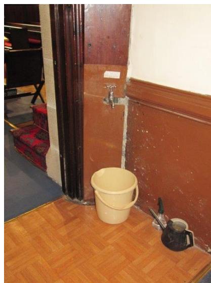
Tap in the vestry with bucket below
