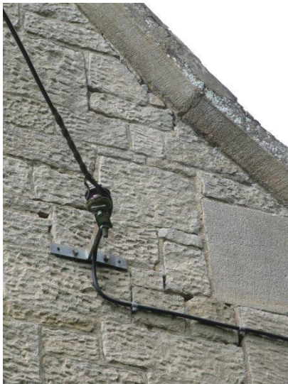
Hungry joints to the Gable
