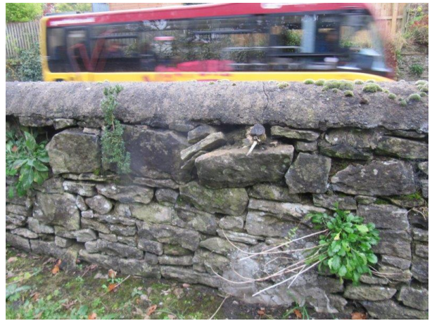
Grass, saplings, open joints and dislodged stonework to the inner face of the Southern Boundary
