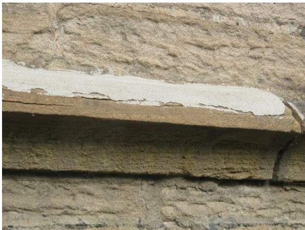
Previous mortar repair to string course on South Elevation
