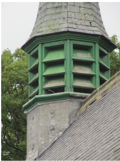
Bare wood visible to louvres on the fleche
