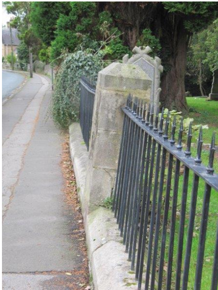
Leaning pier and distorted railing to Southern boundary
