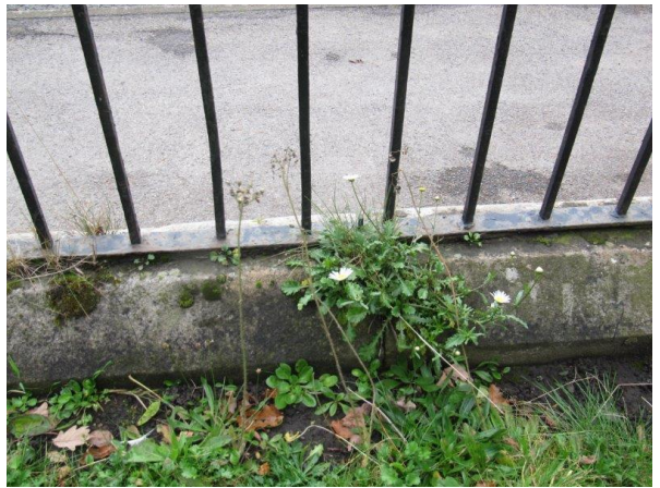
Grass, saplings, open joints and dislodged stonework to the inner face of the Southern Boundary
