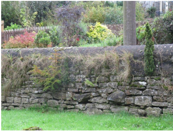
Grass, saplings, open joints and dislodged stonework to the inner face of the Southern Boundary
