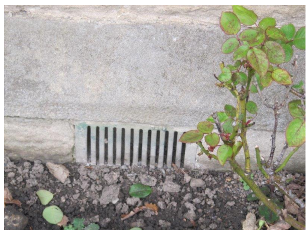
Soil levels close to or covering vents on the South elevation
