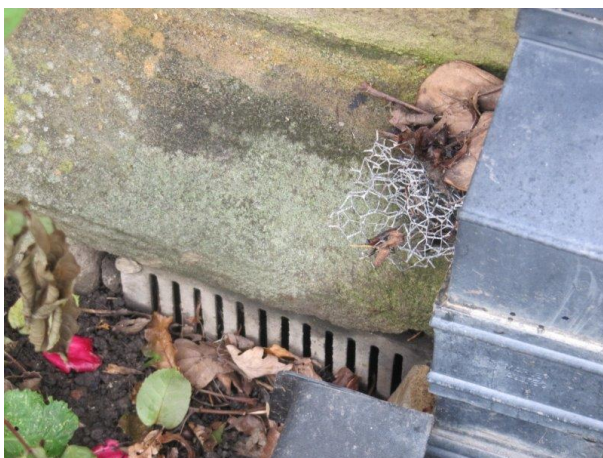
Soil levels close to or covering vents on the South elevation
