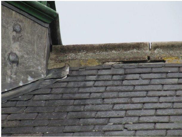
Open joints and failed bedding to main ridge
