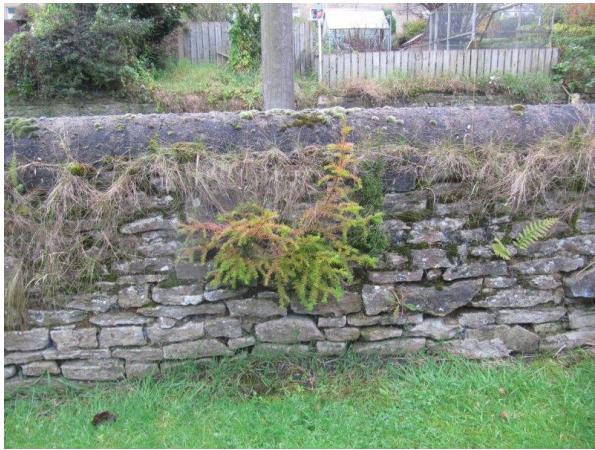
Grass, saplings, open joints and dislodged stonework to the inner face of the Southern Boundary
