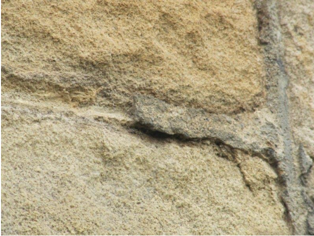
Typical issues with failing mortar experienced around the church
