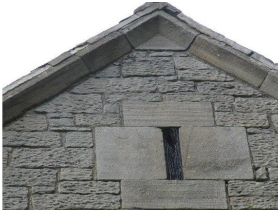
Hungry joints to the Gable of the east Elevation and failing mortar to verge
