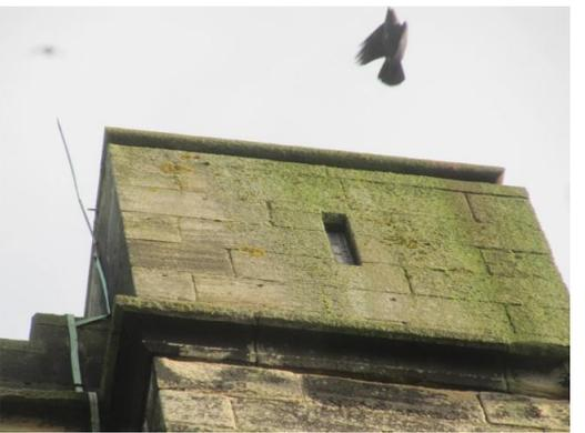
Open joints to the and tower parapet and associated stair turret
