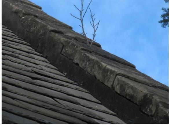
Vegetation and failing mortar fillets to both slopes of the Chancel roof
