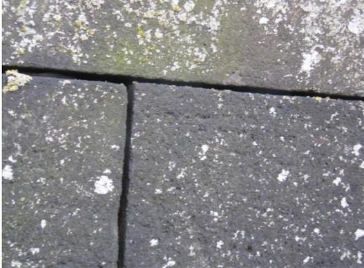
Open joints to the tower parapet viewed internally
