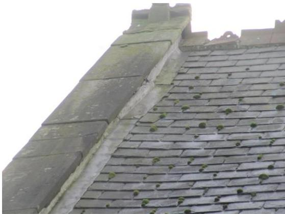
Failing mortar above the flashings and damaged ridge tile to the Nave
