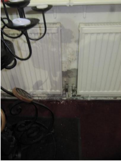
Staining due to water ingress to the South Aisle Plaster failing at low level in the North Aisle
