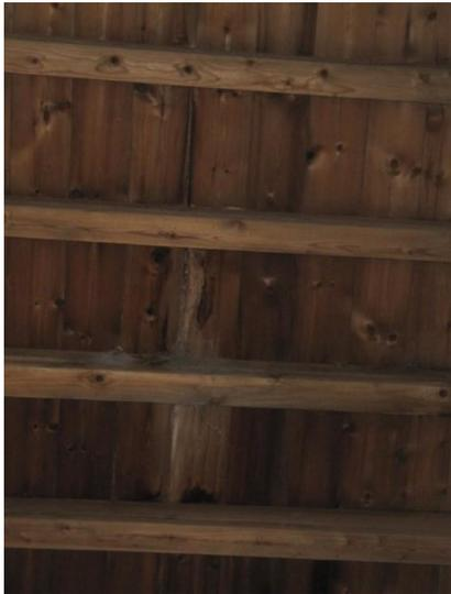
Damp and stained timbers to the tower roof
