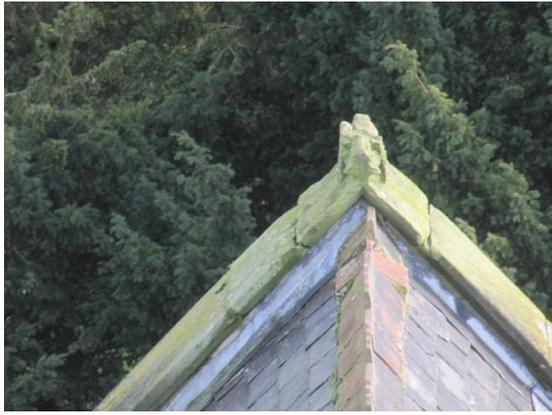
Failing mortar over flashings and damaged ridge tile to the Nave roof
