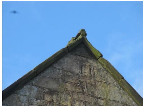
Hungry mortar joints around the apex stone to the East gable of the Nave
