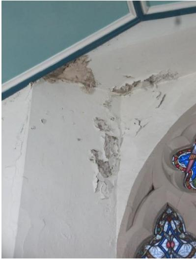
Failing paint and plaster to the East and south walls of the Chancel
