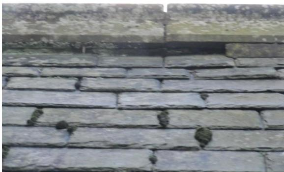
Open joints to ridge tiles and failing mortar bedding to other roofs
