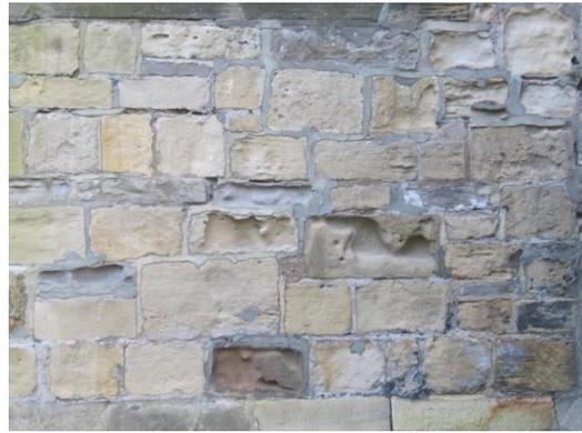
Weathered stonework to the West Elevation of the North Aisle
