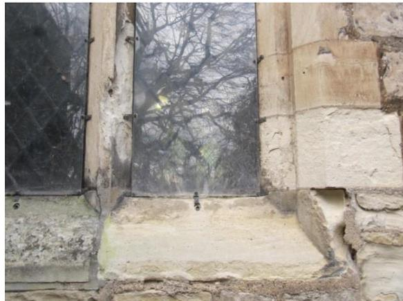
Eroding stonework to the sill and mullion on the South elevation of the Chancel
