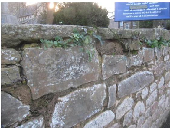
Vegetation growth and failing mortar to both sides of the Eastern boundary
