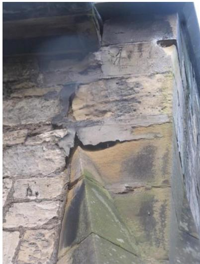
Failing mortar and weathered stonework in the same area
