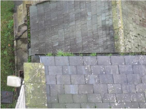
Missing and slipped slates to the North Aisle roof    Vegetation to Northern gutters
