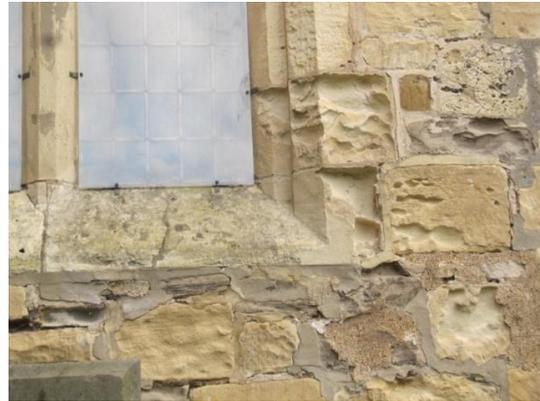
Weathered stonework to the West Elevation of the South Aisle
