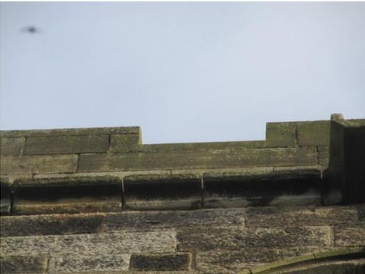
Open joints to the and tower parapet viewed externally
