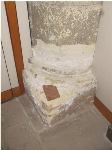
Salts and sanding stonework to the base of the column in the internal lobby
