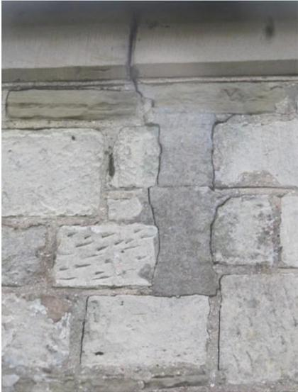
Wide mortar infill showing signs of cracking
