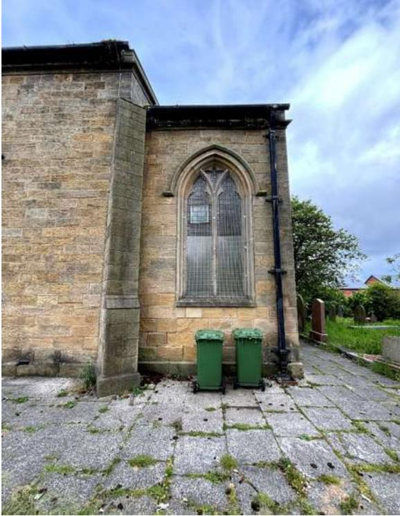
Loss of pointing to lower left side of window and crack to window reopening.
