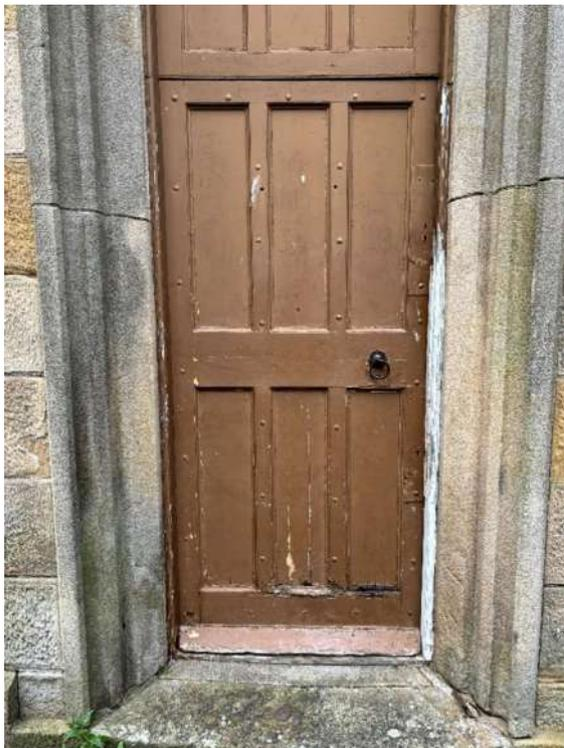
ED.02 showing signs of rot and deterioration to the frame.
