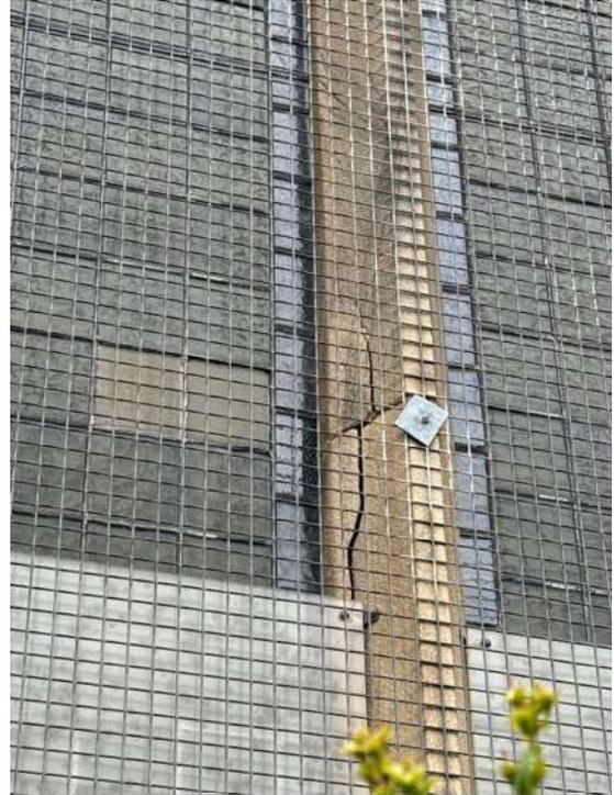
Internally: Cracking to upper left side of paint to mullion.
