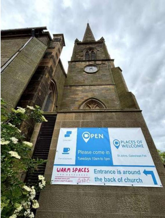
Broken timber louvres, crack to stone ledge and crack to surround of circular opening.
