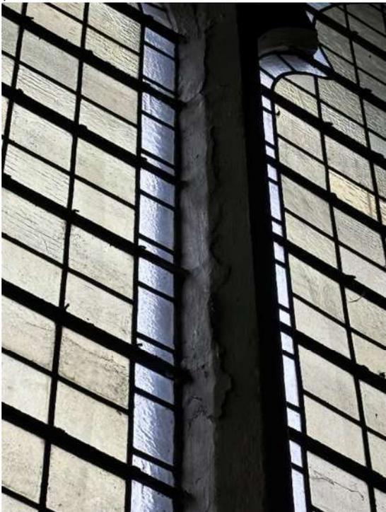
Internally: Cracking of paint to central mullion right hand side and frame.
