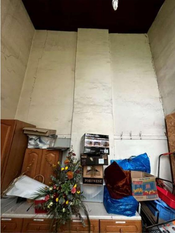
Cracking and flaking of paint to walls and around door.
