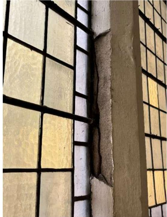
Cracking to paint visible to upper left side of mullion.
