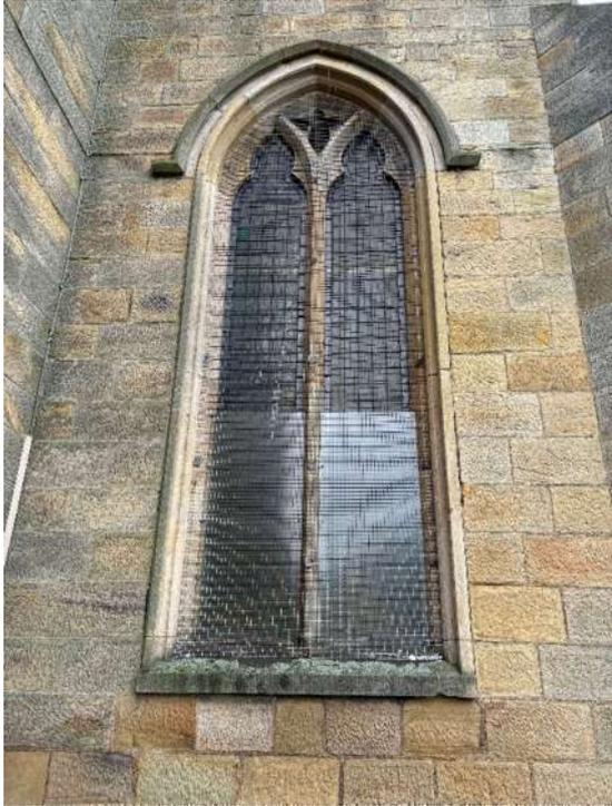
Crack to upper section of mullion, right hand side.
