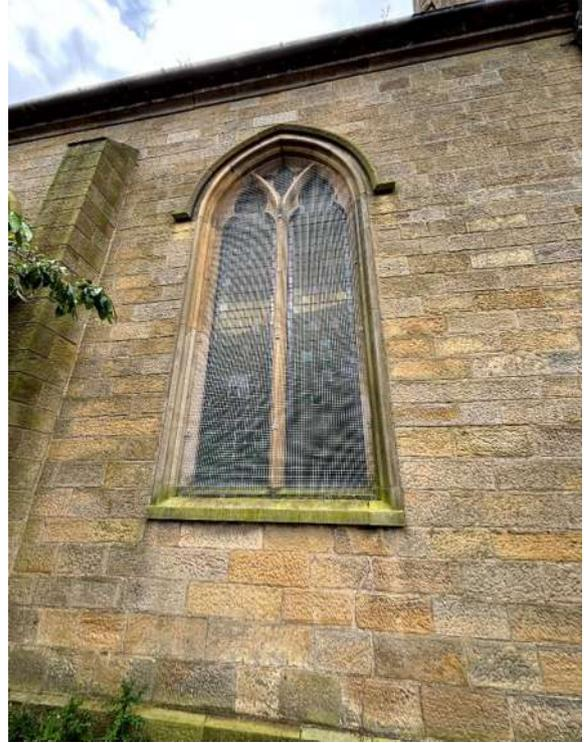
Previously repointed historic crack is reopening with new crack to base.
