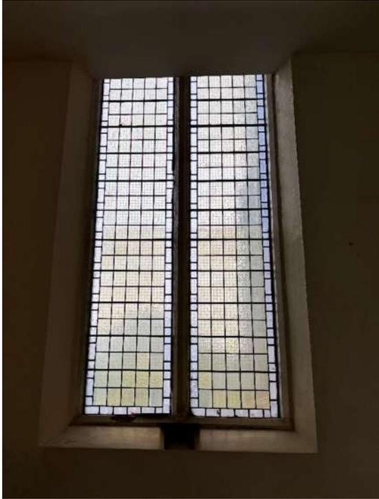
Paint and plaster have fallen from lower left side of mullion, crack to stone visible.
