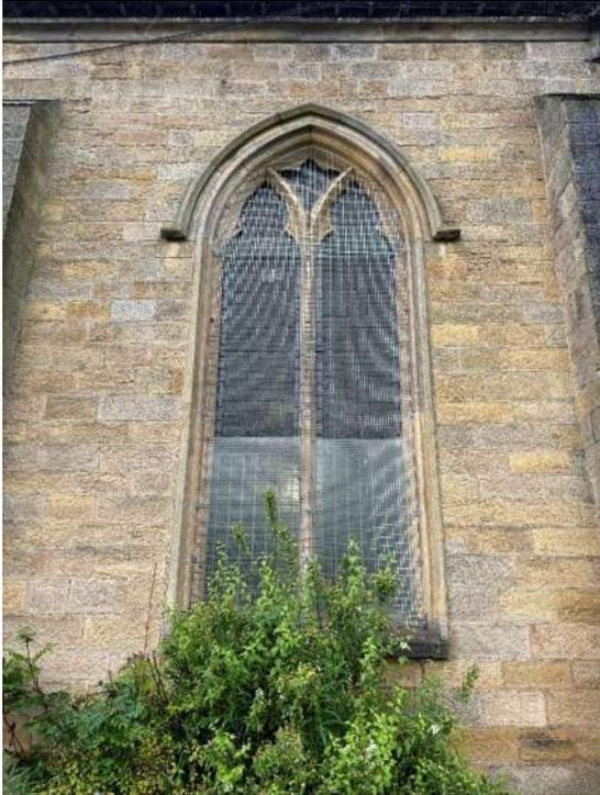
Cracks visible to central mullion left hand side.
