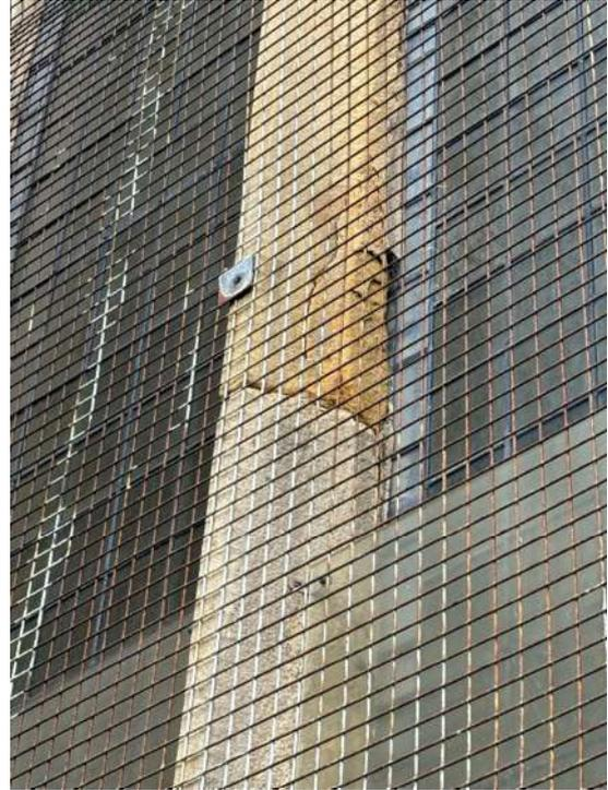
Crack to lower section of mullion, right hand side.
