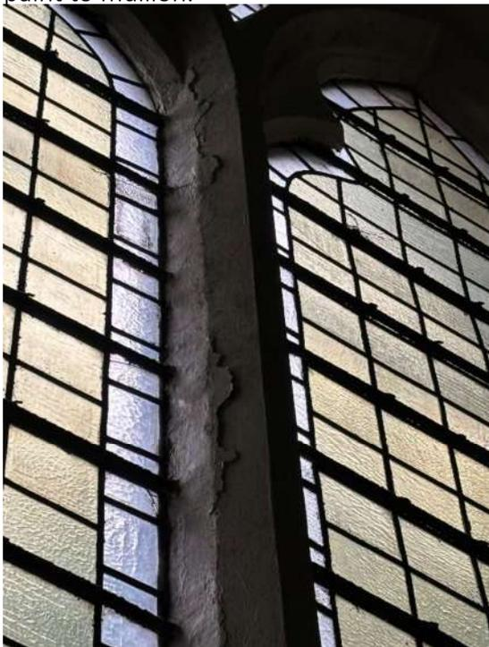
Internally: Cracking of paint to central mullion left hand side.
