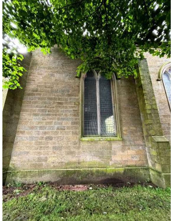
Vent positioned very low into the ground within this bay. Damp evident.
