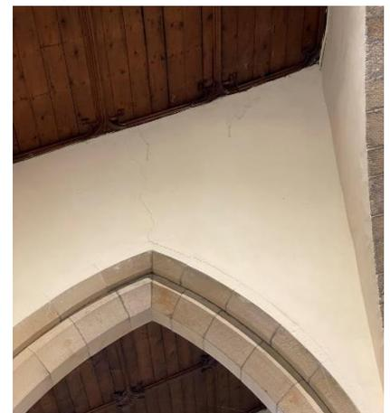
Figure 20- Crack to southern aisle arch
