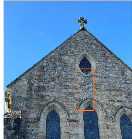
Figure 11 – East lancet cracking
