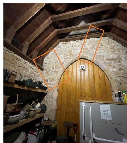
Figure 21- Crack to south porch
