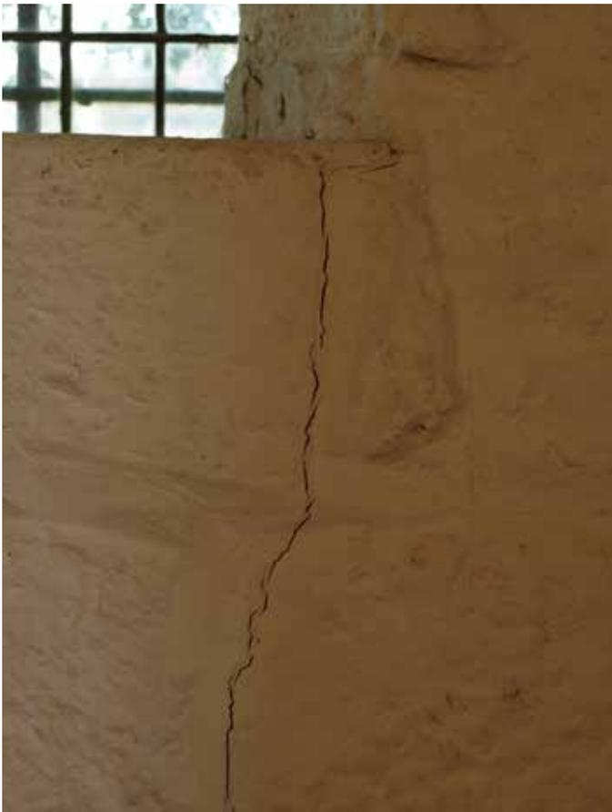
Cracking to the RHS of the East window - through full thickness of wall. Monitor
