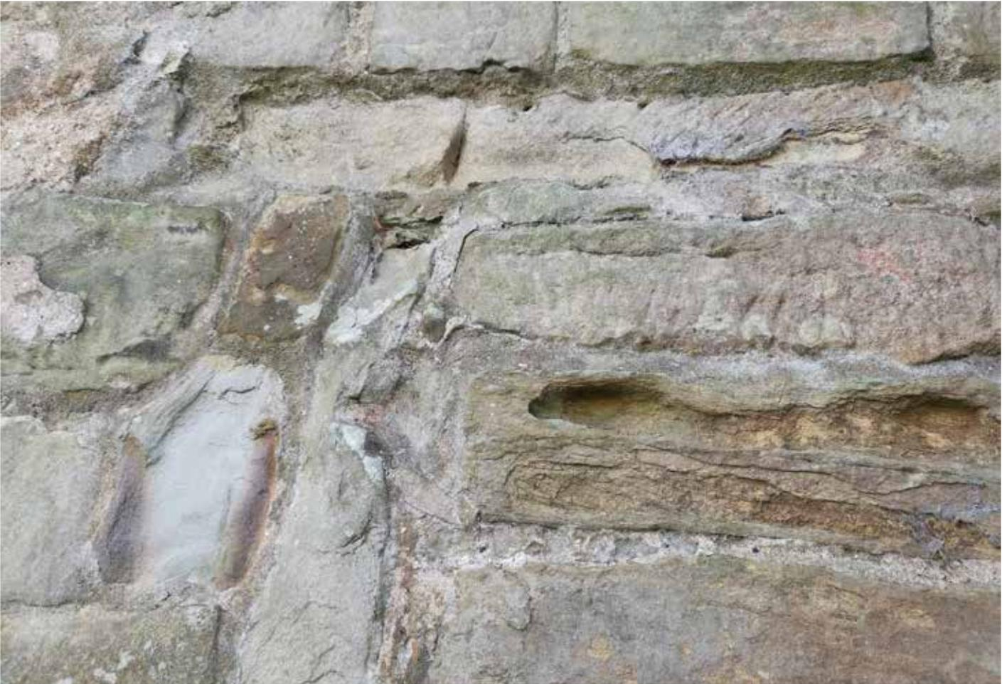
Blocked north doorway to Chancel: deterioration of masonry, in part due to hard cement pointing
