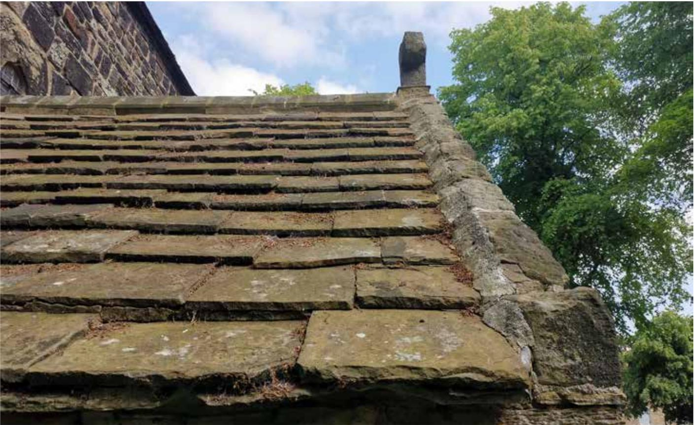
Porch west slope: numerous chipped slates, mortar flashing cracking away from gable
