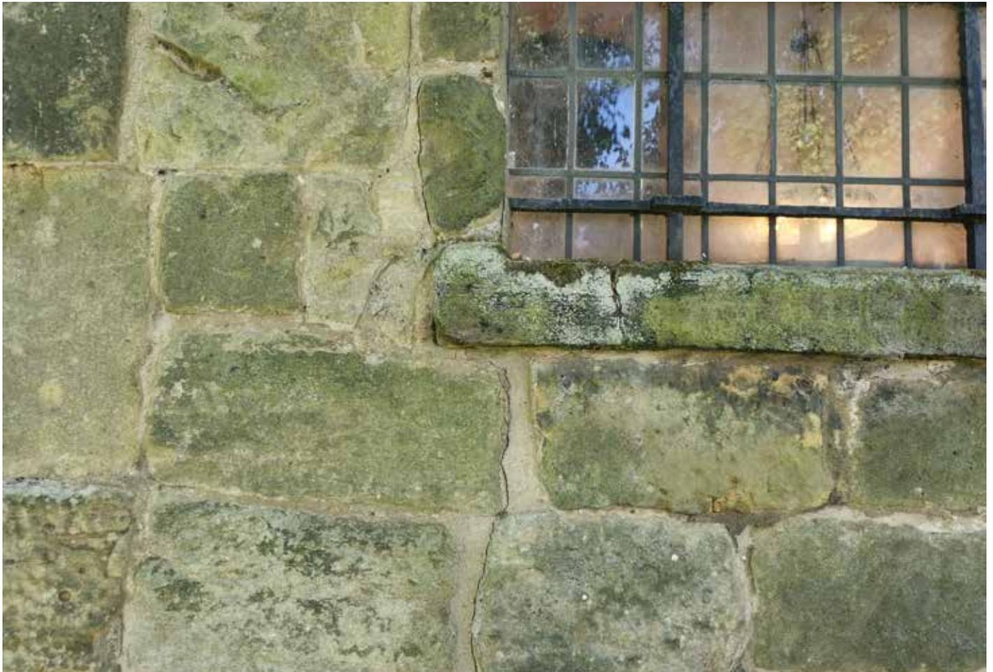
Cracking to East window
