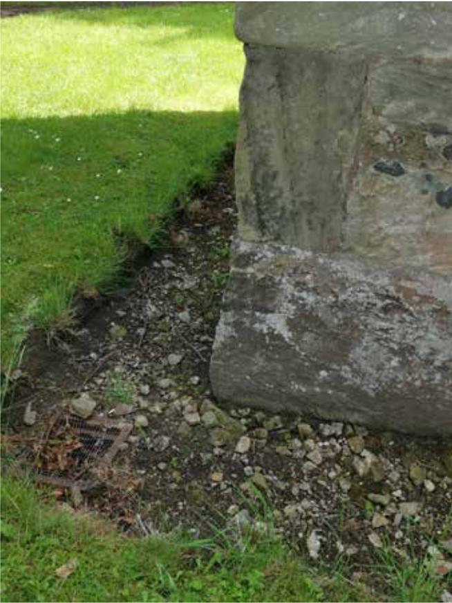
Conditions at the base of the walls are improving now that concrete channels have been removed.
