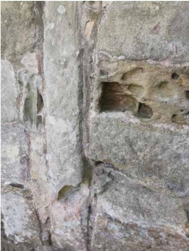
Pockets of erosion to the soft sandstone, isolated but widespread
