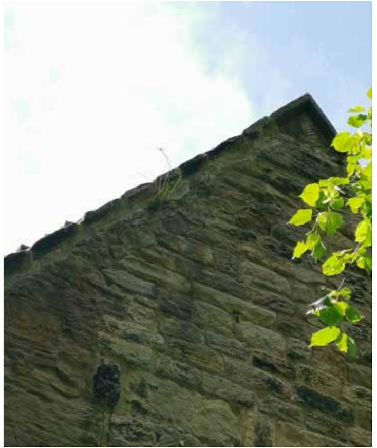
East gable: vegetation should be removed and open joints pointed
