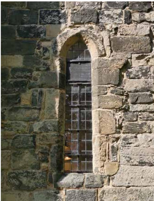
sI: note erosion of surrounding masonry
