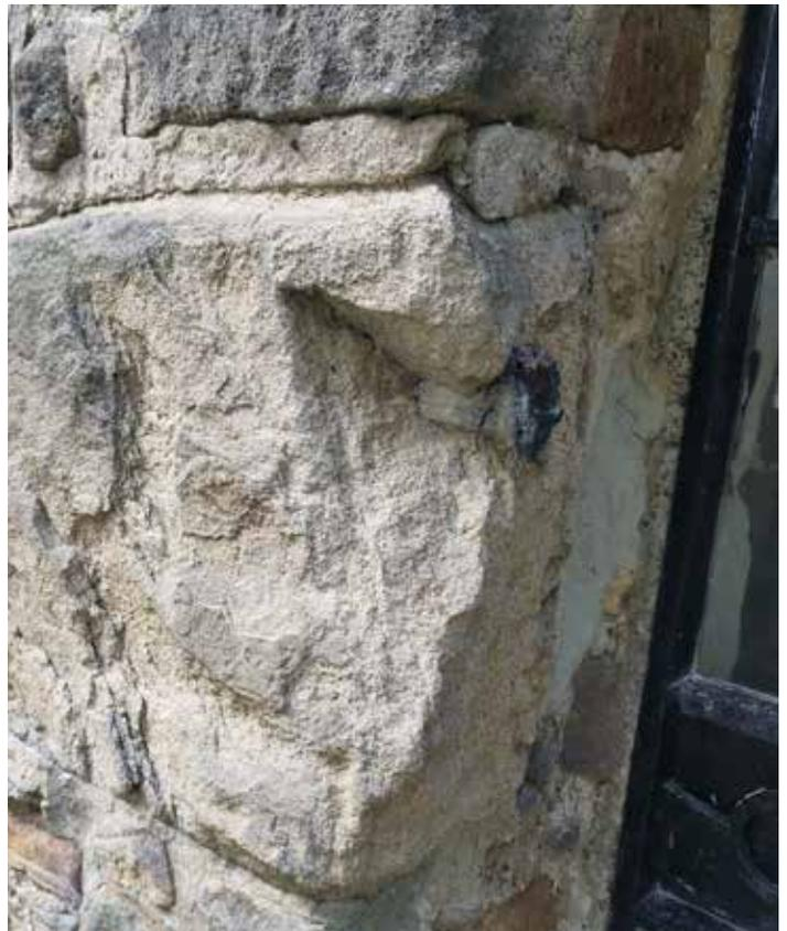
Damaged masonry to jamb of south Porch, due to rusting iron stub (3.07.13)
