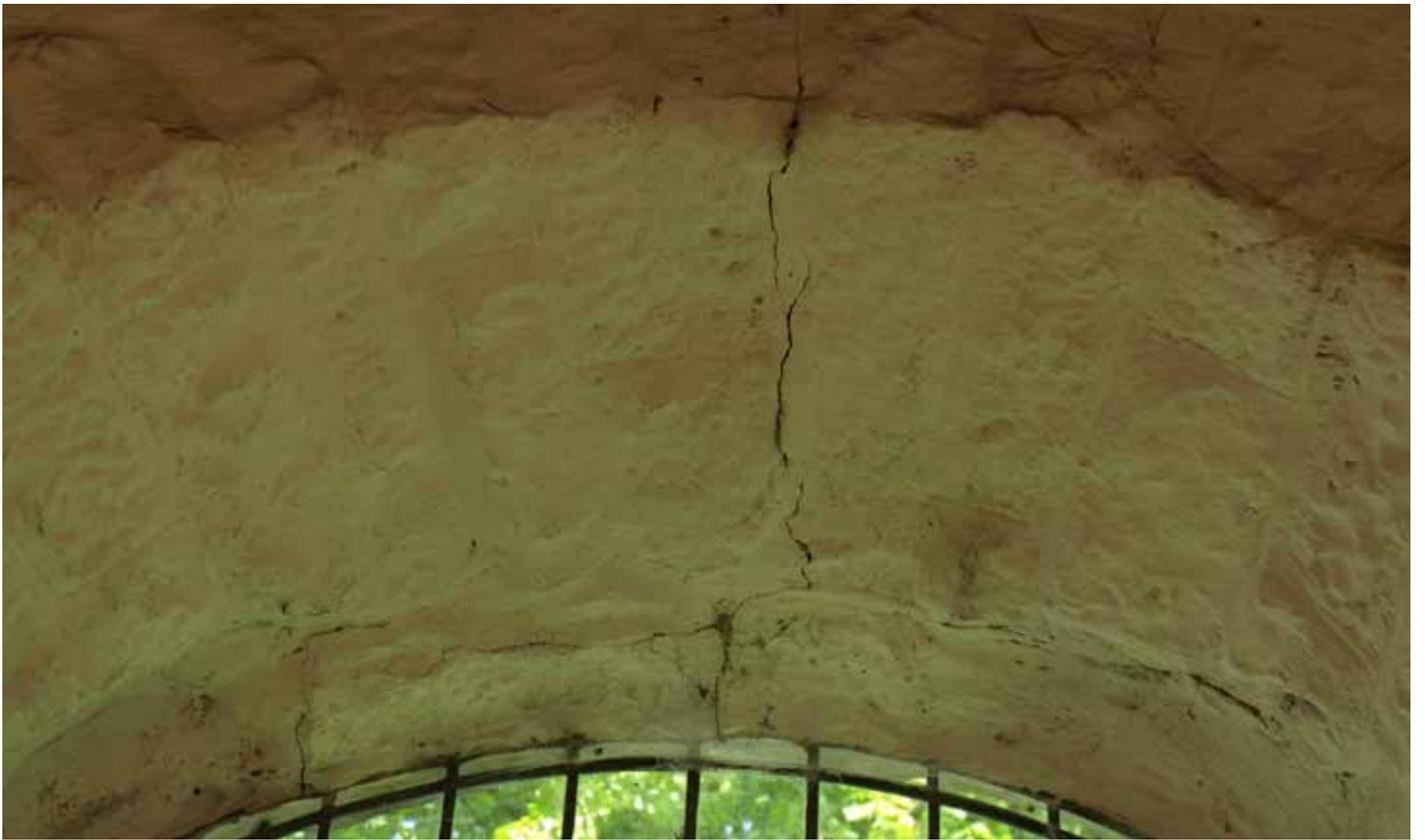
Cracking to head of East window
