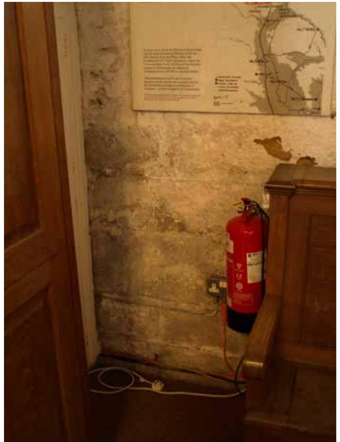
Loss of limewash at low level due to drying of the damp walls. Conditions appear to be improving throughout the church
