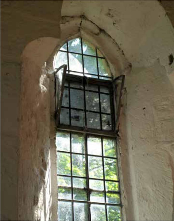
sII: Hopper should be made operational for useful ventilation
