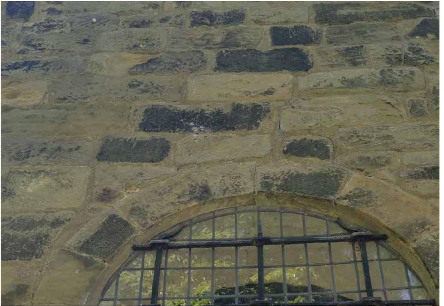
Cracks over head of East window and dropped voussoir (to right of centre)
