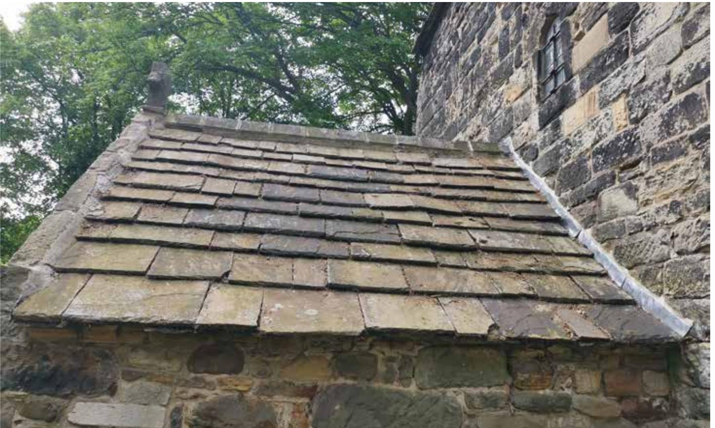
Porch east slope: several damaged slates, mortar flashing cracking away from gable. New flashing in good condition
