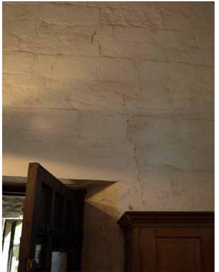
Cracking above lintel to Nave main door
