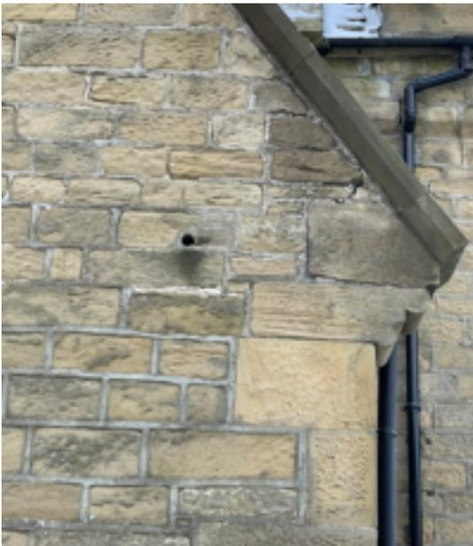
**Vestry north elevation open joints and strap pointing**
