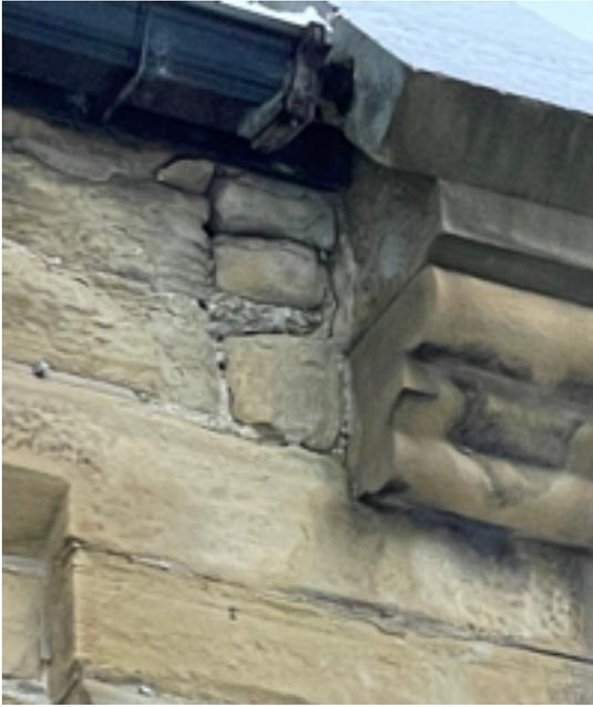
**South elevation east end open joints**
