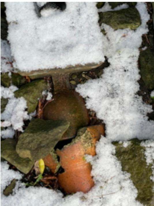
**Sump with broken pipe connection**
