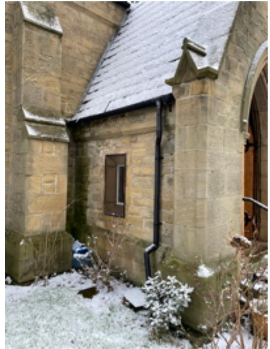
**Porch West Elevation gutter misaligned**
