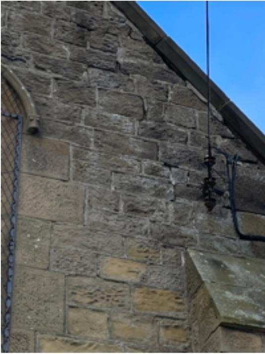
**Chancel east elevation north side open joints**
