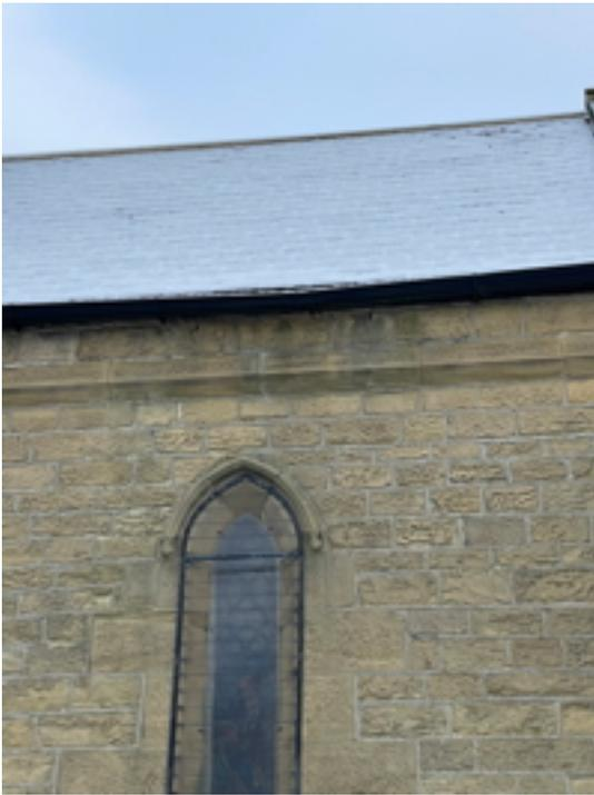
**Chancel South Elevation gutter misaligned**
