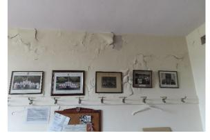
Photo 34, Flaking paint to vestry west wall
