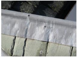
*Photo 3, Example of holes and cracking to lead capping of buttress apex*
