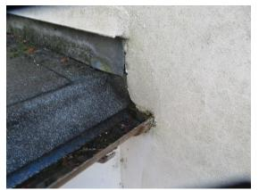
Photo 9, Gap between flashing and roof felt upstand
