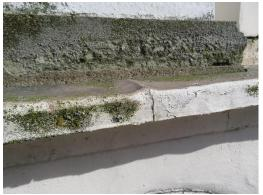
Photo 24, Crack in lead to statue base
