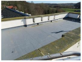
Photo 7, New plastic roof membrane to tower roof, gaps in the pointing to the coping stones.
