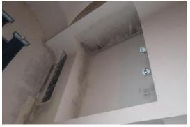
Photo 30, Example of mould to ceilings and walls
