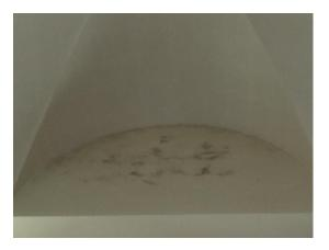
Photo 33, Mould to arched sections between frames
