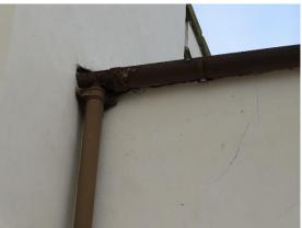
Photo 10, Displaced gutter joint
