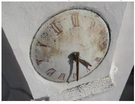
Photo 23, Deterioration of finish to clock face
