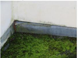
Photo 8, Example of slipped flashing over flat roof interface
