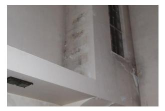
Photo 32, Cracking, mould and discolouration to NE corner
