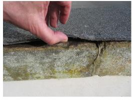
Photo 6, Lifting felt to Vestry parapet
