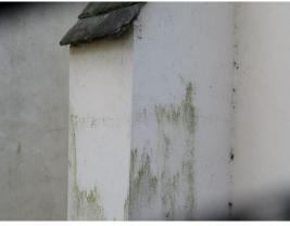
Photo 17, Regular spaced cracking to render on buttresses visible externally and internally
