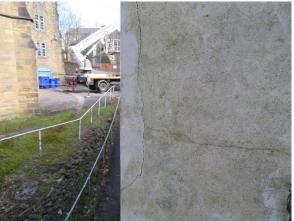
Photo 15, Example of vertical and horizontal cracking on buttresses
