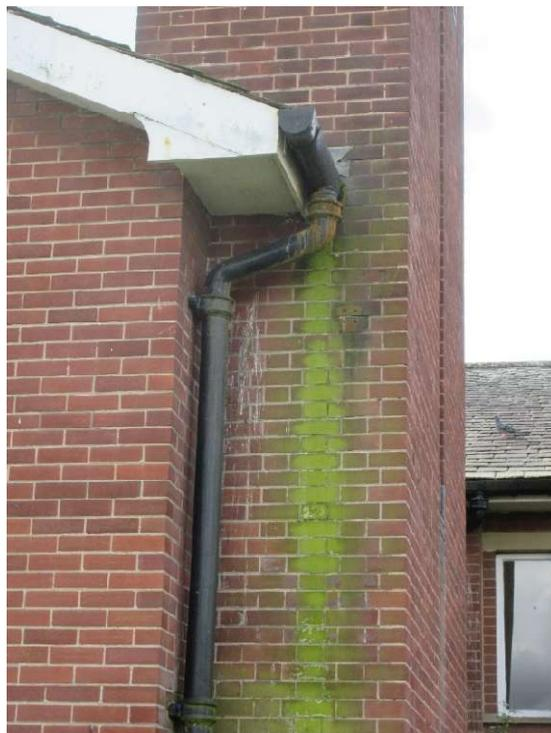
17. Small pipes from the Tower top gutters turn into the brickwork and out again into its back gutter. Holes through the bricks inside the cut out cross allow access to the internal rainwater pipe.
