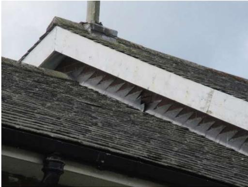
loose flashing unchanged since 2018
