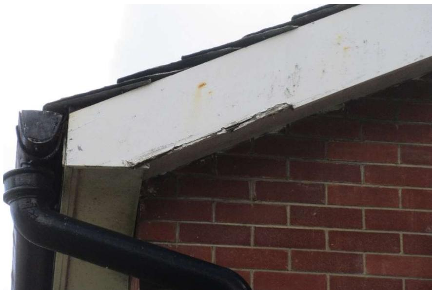
Minor decay of bargeboard where swept timber cover missing at NW Nave
