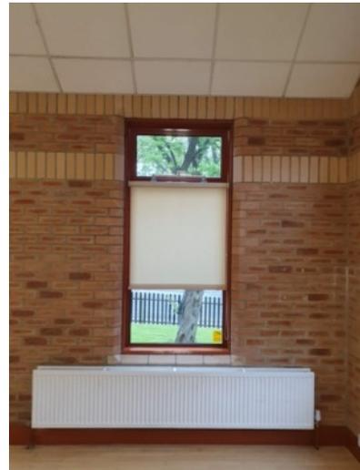
b) Facing brick internal finish with typical window detail
