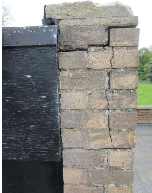
Details of the coping and parapet brickwork at the end of Stair (top left in photo below)
