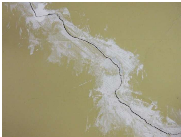
Old cracks outside and inside Hall W corner
