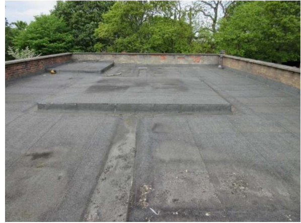
Ponding at deflection of deck at Hall SE
