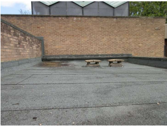
Roof over vestries, ponded in corner over lobby, movement joint against Church wall
