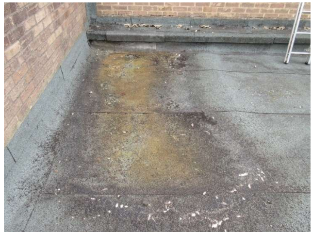
Roof over vestries, ponded in corner over lobby, movement joint against Church wall
