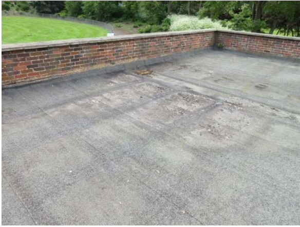
Ponding at deflection of deck at Hall SE
