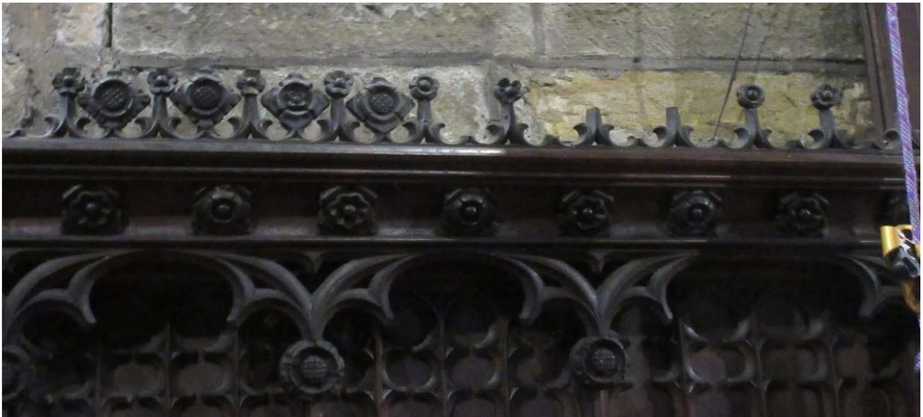
92. Dado panelling along S Aisle wall may be reused box pews. Good condition except worm holes and a small gap and split in the panelling E of the Porch door where most worm. May have been treated so to be observed for fresh dust (suggesting new emergence) in early summer.
