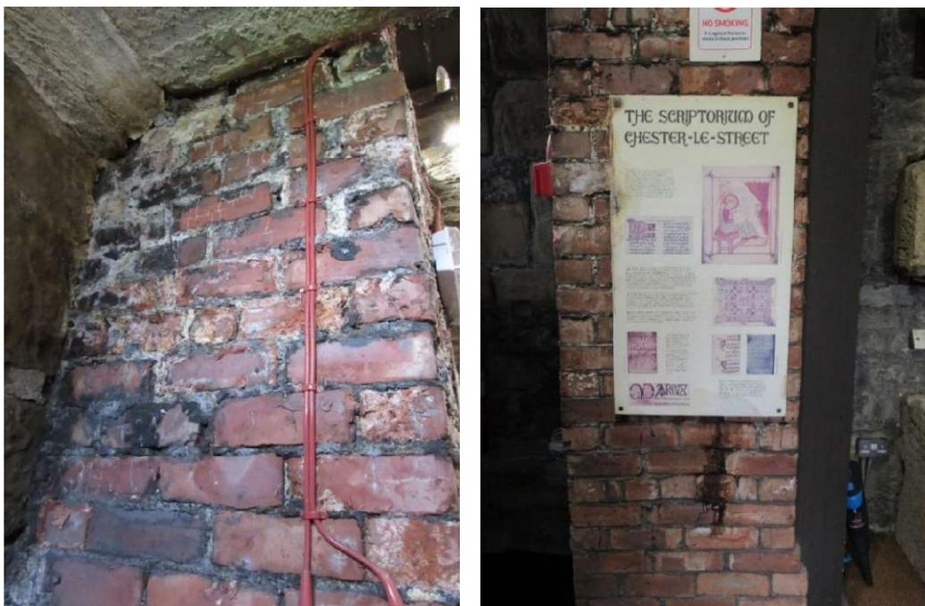
Brick Chimney where it passes through the Ankerage salts continue to effloresce full height especially at top and now tarry water seeps out at head height
