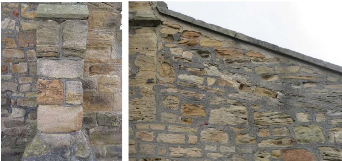
43. Ankerage W, N side – good except a few pocketed stones at upper W side and next to buttress which might be filled with soft lime mortar to slow decay.
