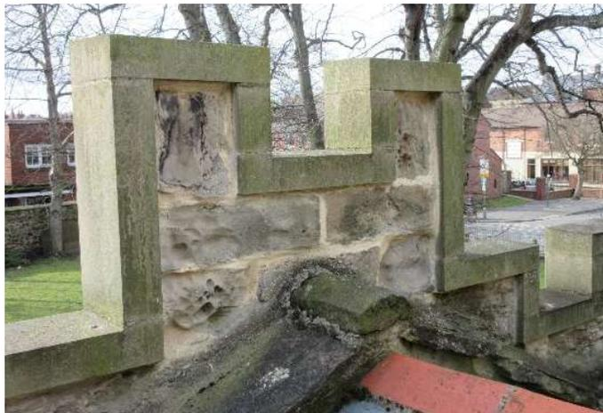
42. S Aisle W gable including its N buttress – many stones including the buttress have slight surface decay behind hard dark pointing. Scattered pocket decay especially close to the top of the gable.
