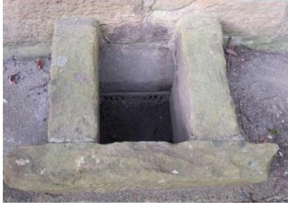
110. If the floor under the Organ remains suspended timber, prevention of rot depends on the small rusting grating through the Organ N wall.
