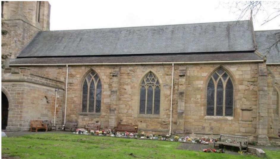
40. At SE a curious small rectangular frame with decayed moulded head and sill and one missing side around a blank panel. May be best removed and infilled to match wall.
