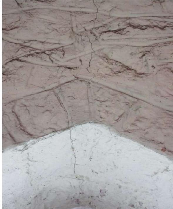
34. The tops of the arches at three external windows have hairline cracks, widest at N where at most it is 2mm and extends into the wall above.
