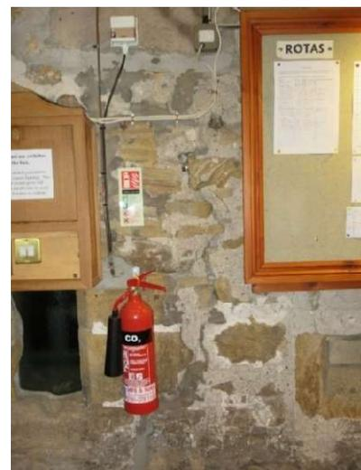
88. Remaining walls mixed stone sizes and pointing materials. Fair but some parts dirty and dull due to dark cement pointing. Choir Vestry (former Porch) walls bare ancient masonry mainly hidden by cupboards.
