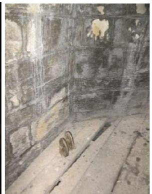
Stainless or galvanised top lattice typical timber platform of mixed boards and beams with sand debris & loose boards
