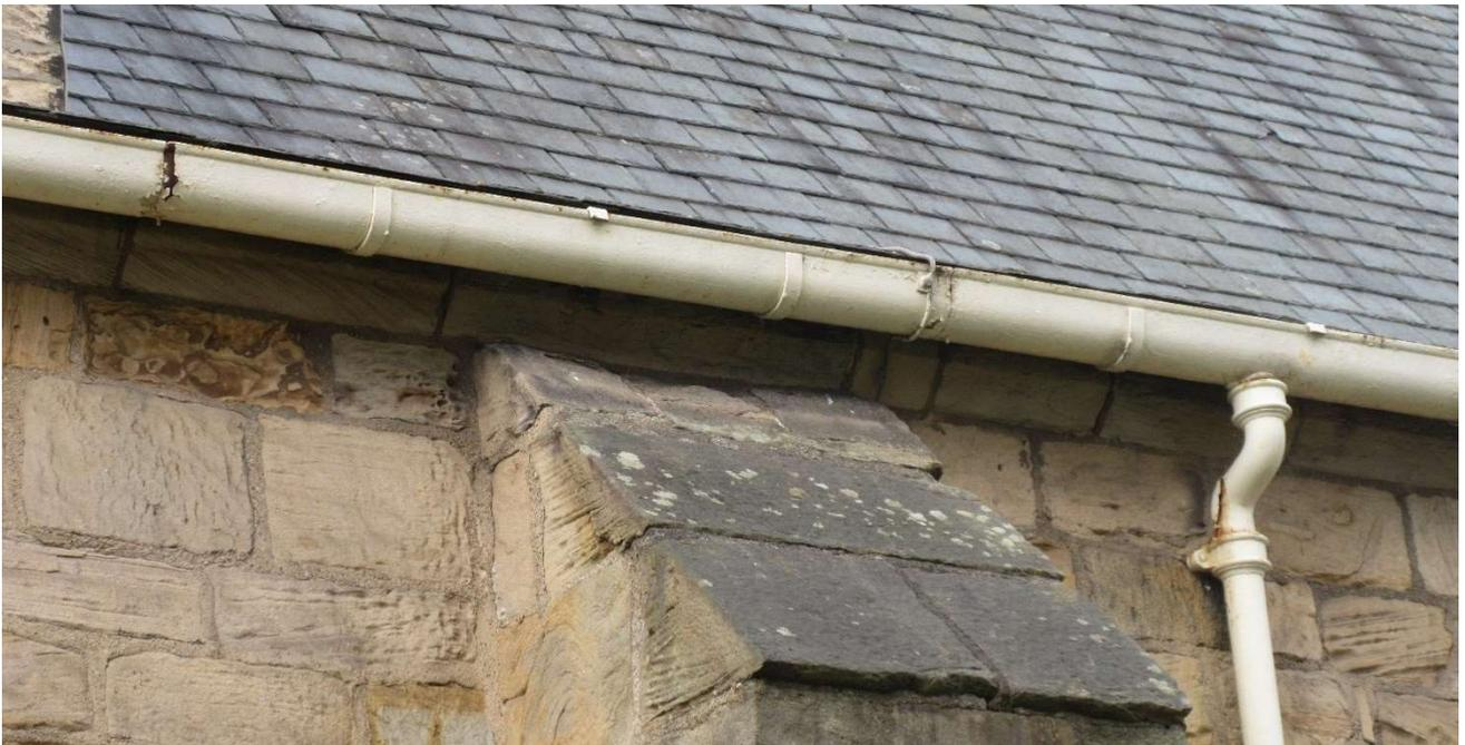
S Aisle W end – gutter and pipe breaks
