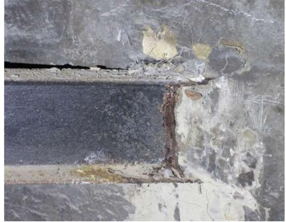
Rust begun at a clock steel embedded in the spire shell
