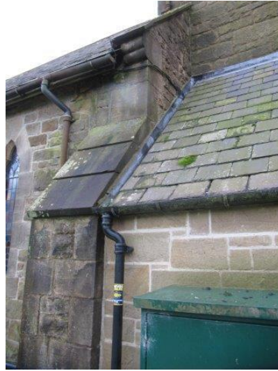
Buttress to West of Nave
