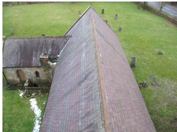
General view of main roof looking East
