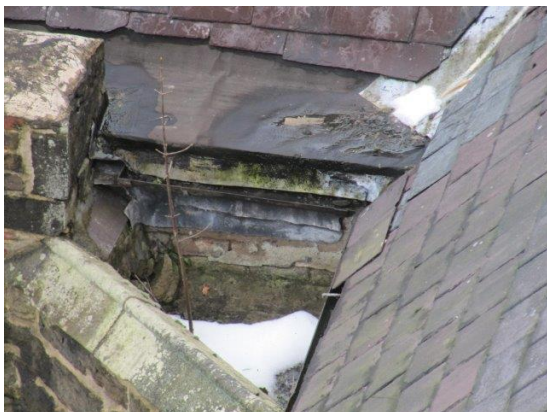
Close up of area over angled stonework between Nave and Vestry
