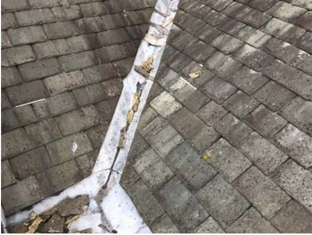
Photo 14: Patched lead gutter and mortar pointing over Narthex
