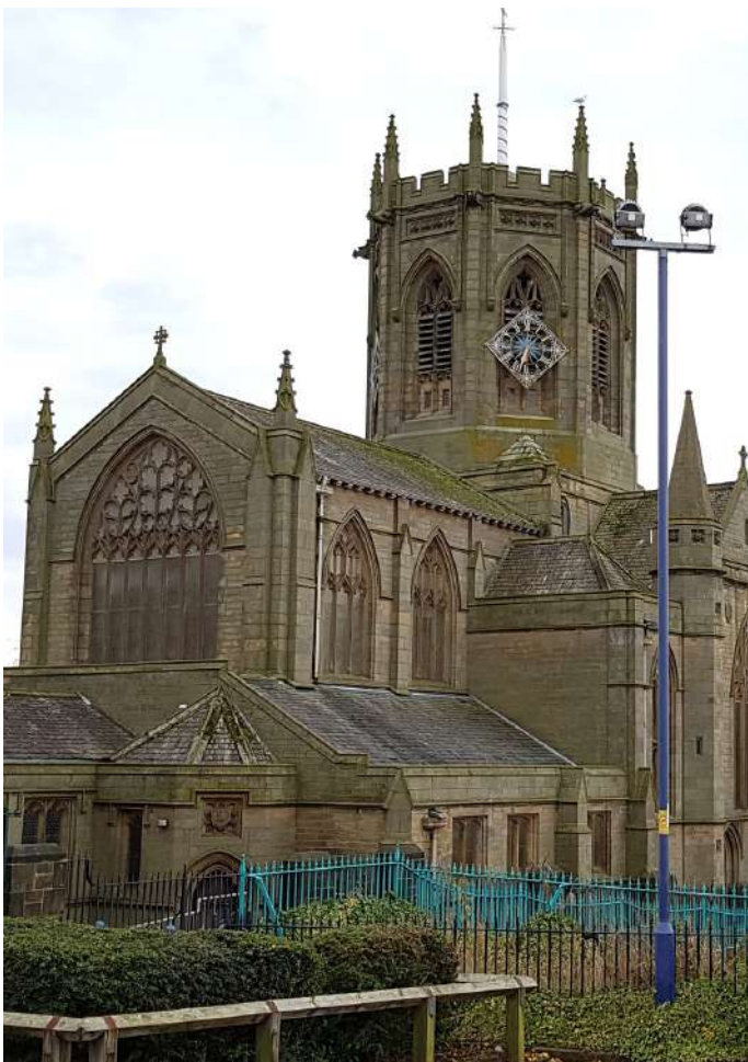
Remaining roofs generally in poor condition with many missing, cracked and broken slates - slates at end of life
