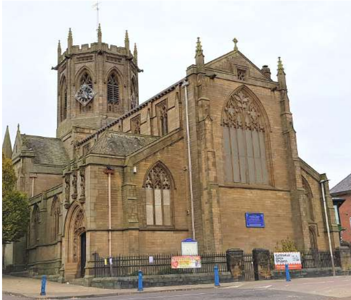
Upper section of west gable (above window), and western faces of octagonal tower were re-pointed in 2015
