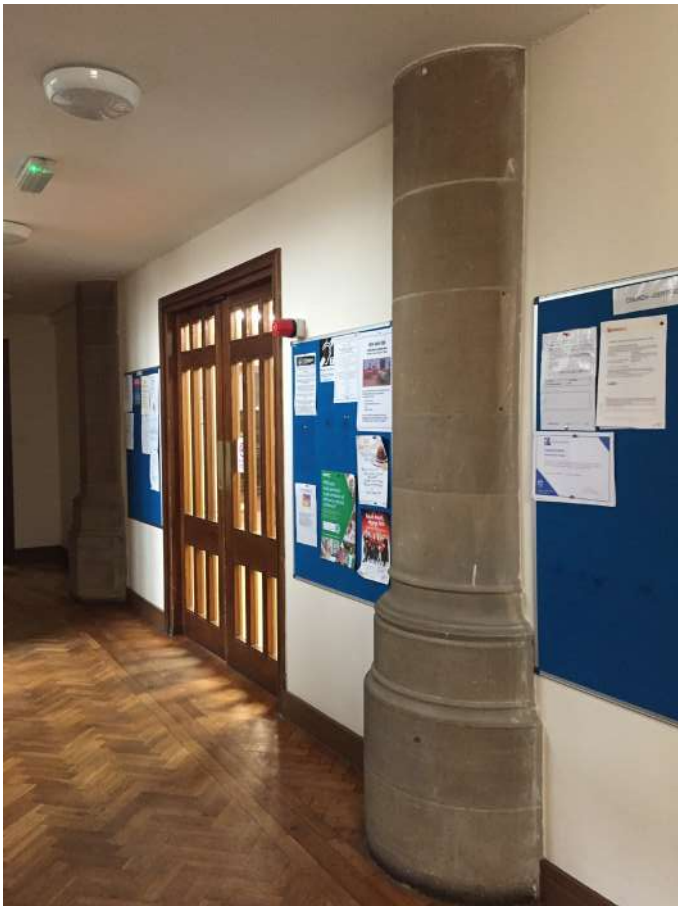
Entrance into community hall from former north aisle
