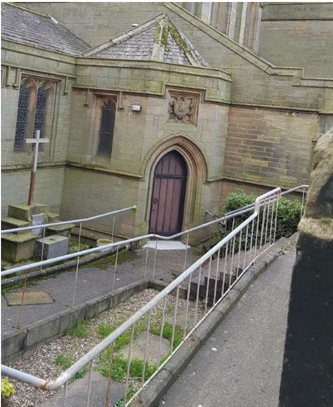
Accessible ramp down to clergy entrance at north-east end of church - not idea for access into community hall
