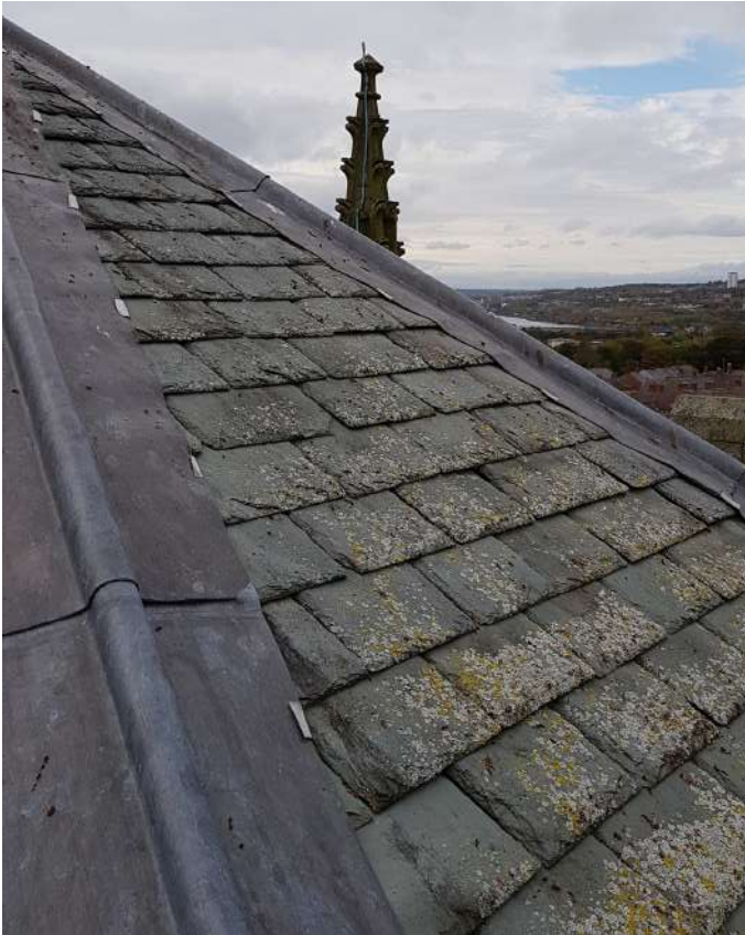
Tower roof re-roofed in 2015, in excellent condition
