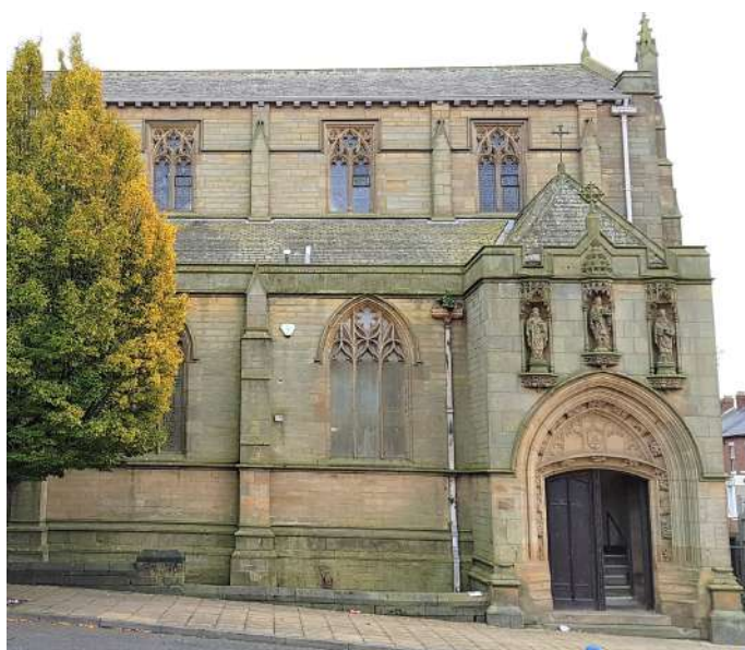
High-level nave eaves gutters, hoppers and downpipes all refurbished in 2015. Rest of rainwater goods require refurbishment during roofing works
