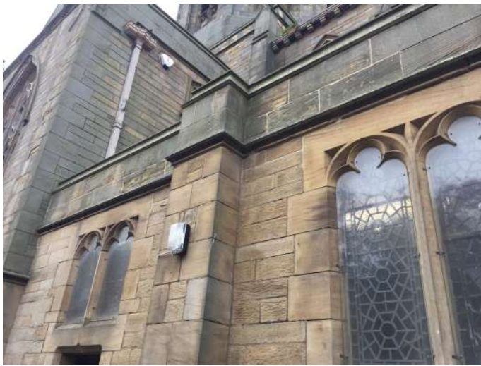
Parapet over southern garden door re-pointed (south chancel aisle)
