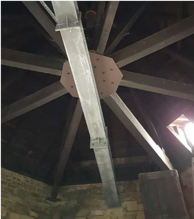
Modern steel support to roof - no movement noted
