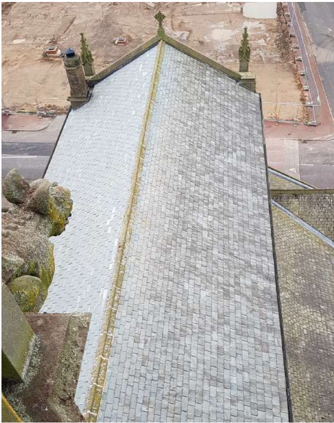
Nave roof re-roofed in 2015
