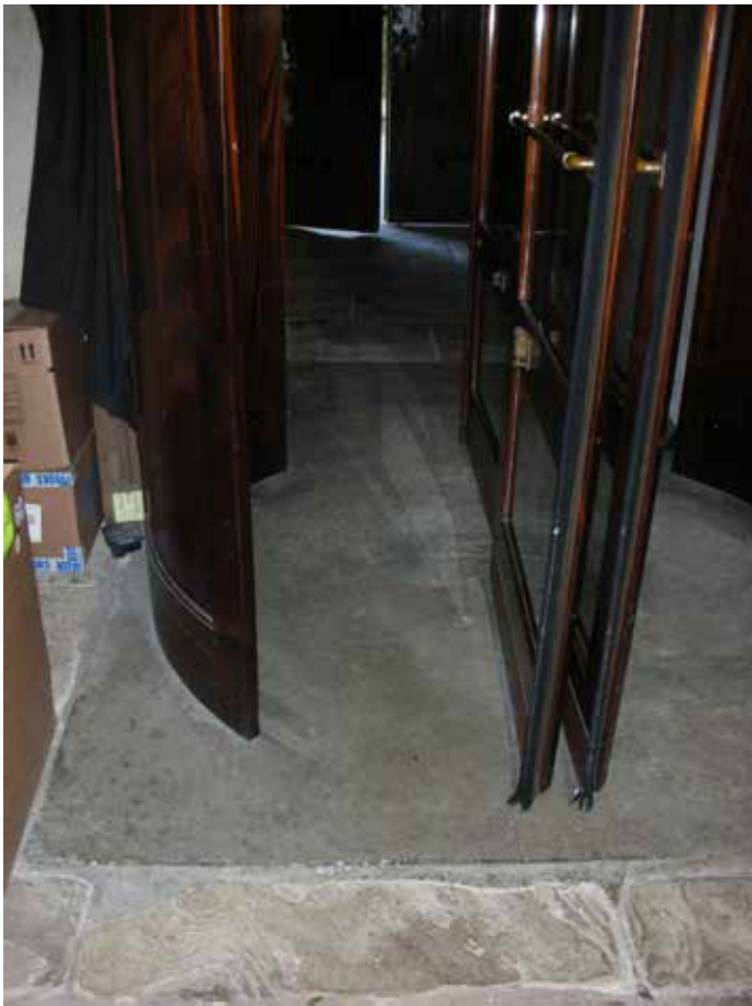
Screed over stone flags to west revolving door
