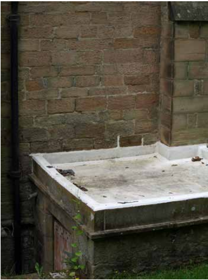
Recent new roof covering to redundant organ blower room
