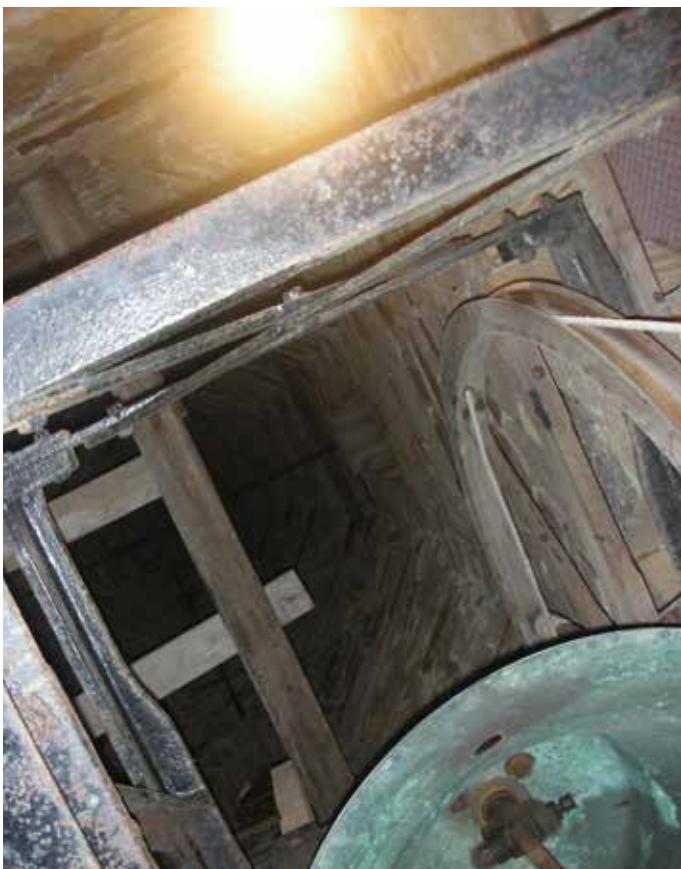
Stonework of spire seen through bell frame
