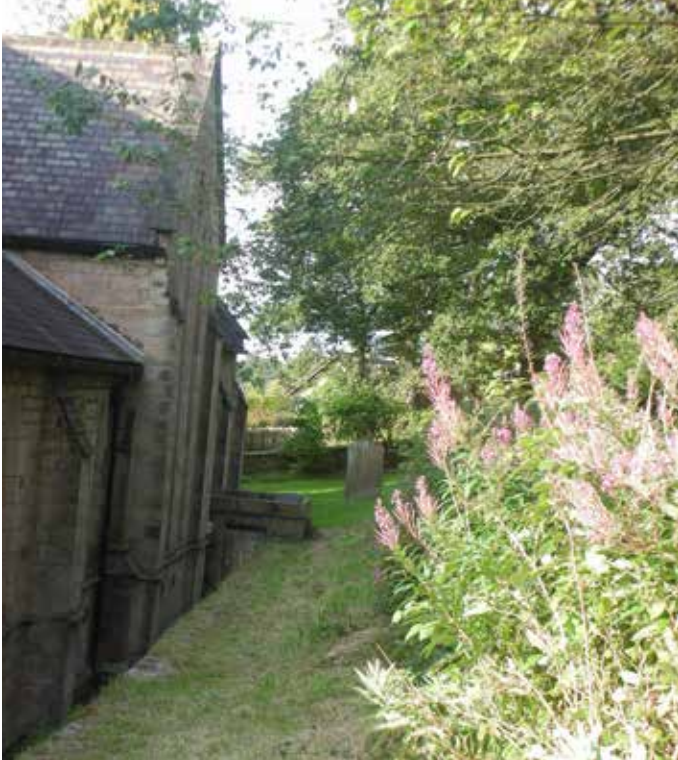
Liturgical south side of church, on top of retaining wall
