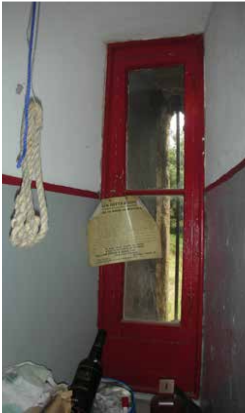
Right: Glazed internal windows in bell ringing chamber
