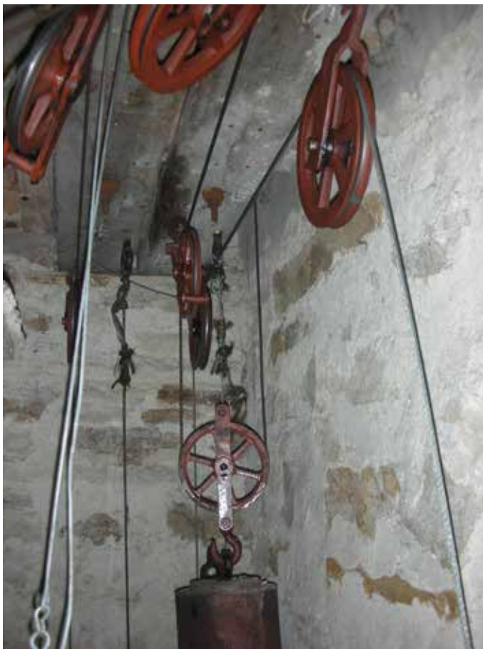
Stonework with rough render to clock chamber
