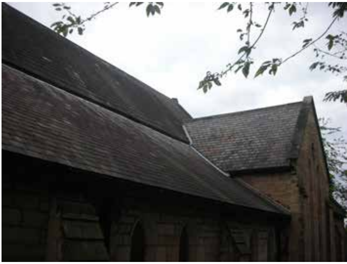
South roof pitches of nave, south aisle and south transept
