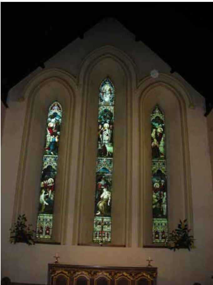
Main east window - all glazing in good condition
