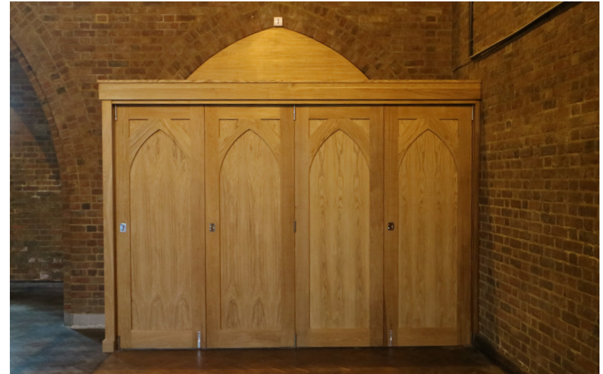
View of oak infill to arch and concealed tea station within oak cupboard
