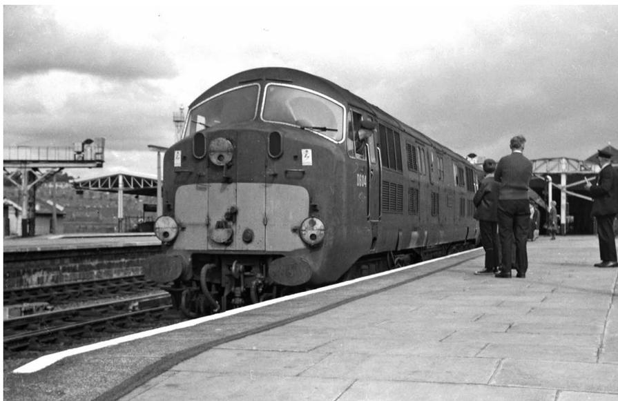
*D604 Cossack was one of the very first batch of WR 'Warship' diesel hydraulics and is seen here at Plymouth in late August 1965. The entire class was withdrawn by December 1967.*
