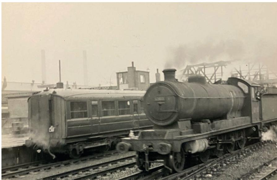
*Also seen at Doncaster on 1/4/1961 is a southbound freight with a Cl. O4/8 2-8-0 engine as motive power. By this date these rebuilds with Thompson boilers constituted the majority of the class.*
