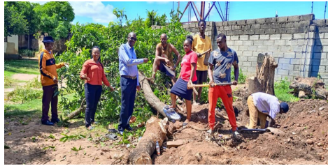
Members of St Paul's, Chipata South laying new school foundations.
