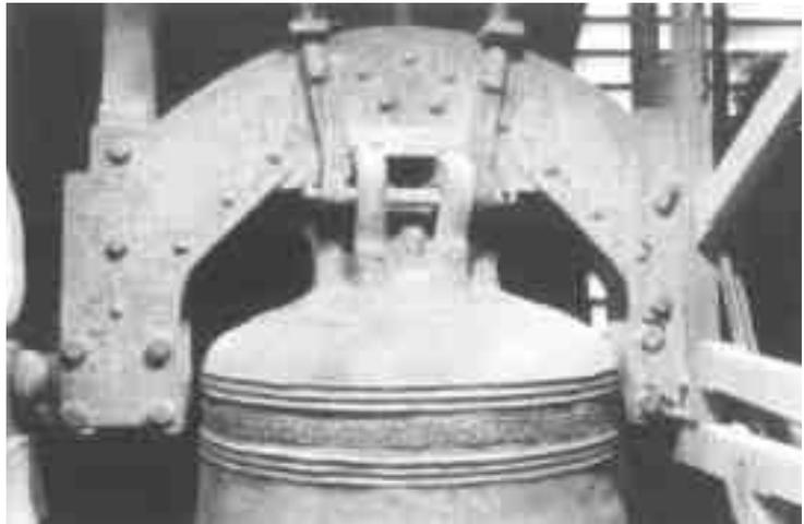
Where fewer than six canons remain and there are no holes through the crown, 'U' bolts may be fitted around the surviving canons and that part of the deadstock or headstock over the stumps of the broken canons extended to butt on to the crown.
