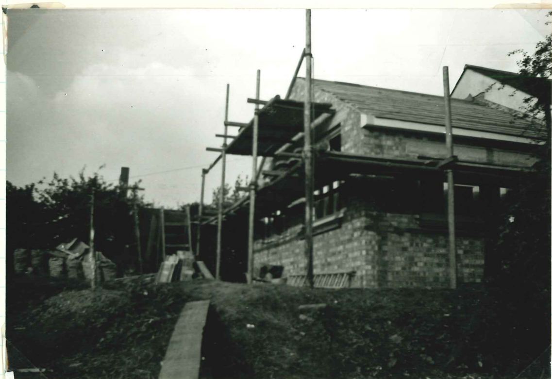
MINOR HALL, SIDE VIEW. (NO FIRE STATION!)
