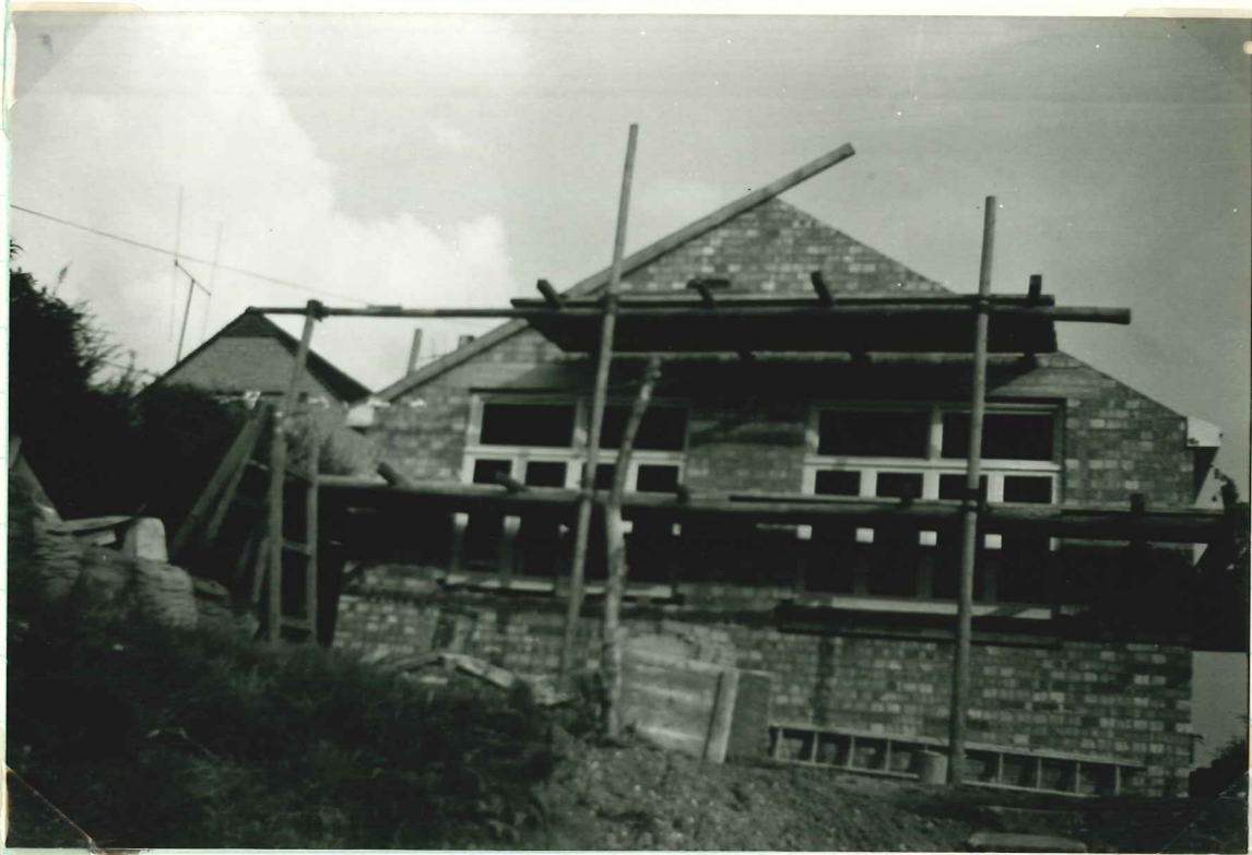
THE MINOR HALL UNDER CONSTRUCTION,
