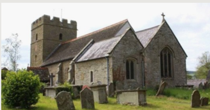
St Swithin's, Clunbury
