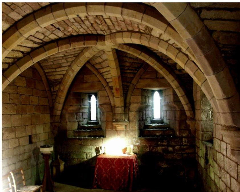
Five steps lead down from the south door to the slabbed floor of the main crypt chamber, which has a groined vault in two bays; the NCH (107) describes it as being ‘a peculiar combination of the quadripartite and sexpartite forms, the outer halves of each bay being of the latter, which the inner, where they conjoin, is of the former construction. The transverse rib is semi-circular’. The vault ribs are all chamfered on their lower angles. Three lancets that light the crypt -
