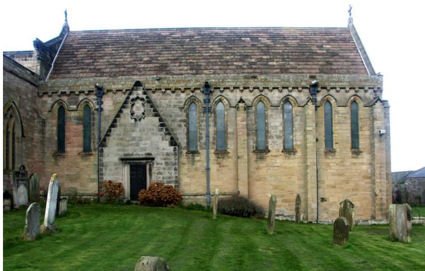
The **Chancel** is constructed of yellowish coursed squared stone; there has been extensive restoration and re-facing. It is five bays long, and has a large plinth with a bold roll at the top and two chamfered steps below. The second bay from the west was remodelled in the early 19<sup>th</sup> century, and has a priest's door set in a shallow gabled projection, of grey
