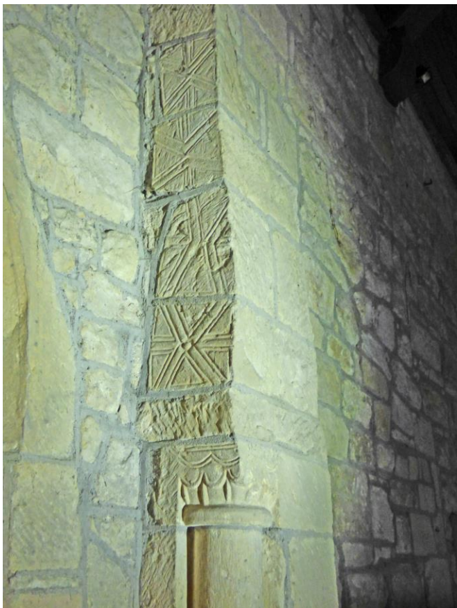
Remains of Sanctuary Arch (on north)
