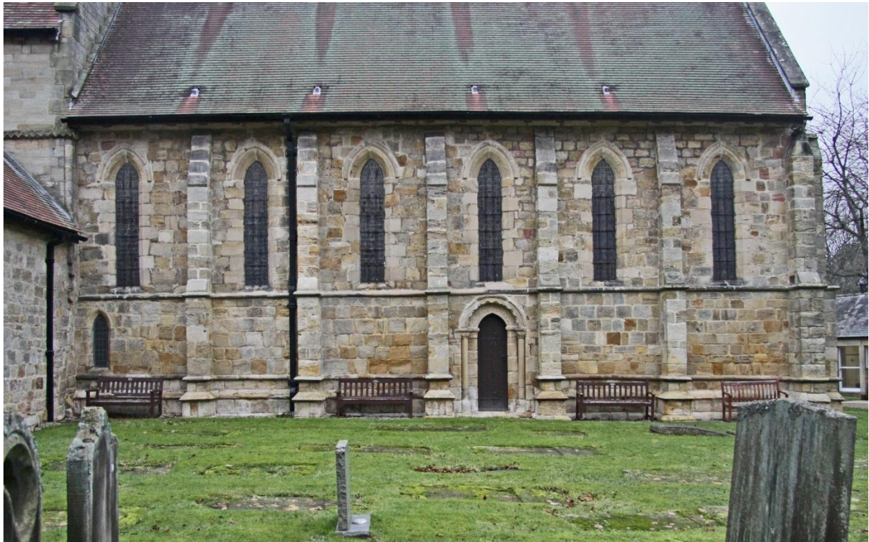
The chancel from the south
