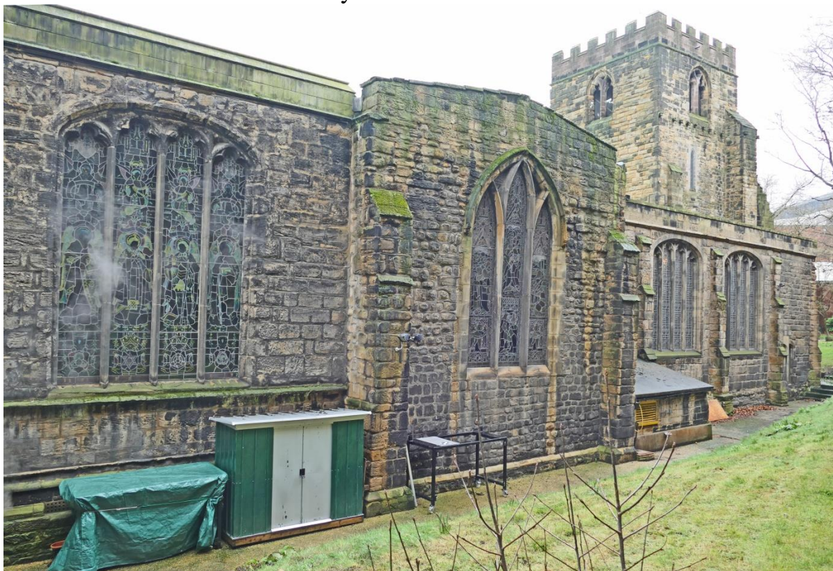
The church from the north-east; note different levels of footings
