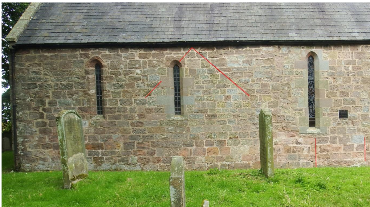
Chancel and west part of nave seen from the south. Highlighted in red the roof-line of the 1839-1893 south porch, and the jambs of the medieval south door
