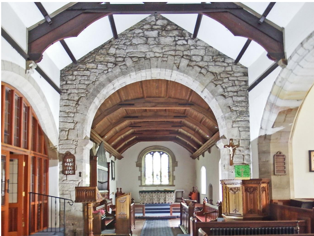
Interior looking east, showing the chancel arch
