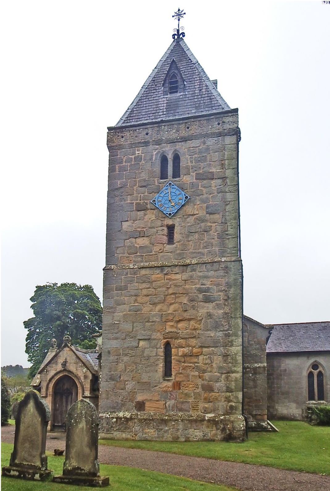
The tower from the west; there is little sign of the former west door removed in the 1850s (bar the line of its porch roof, on either side of the restored lower stage lancet). Note the range of probable gunloops in the parapet.
