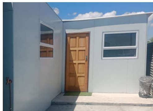
Illitha Pre-School external improvement
