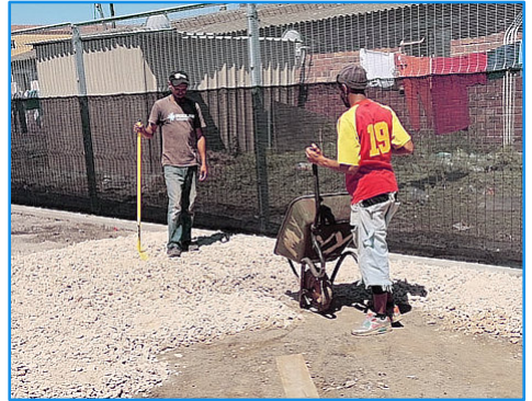
Levelling the uneven play area surface in preparation for artificial grass.
