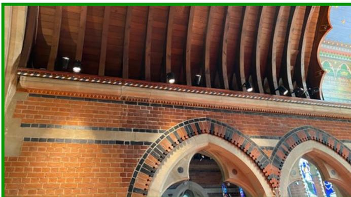
We envisage that a creative lighting scheme combined with a lighter floor and furniture will lift the ambient light level to between 50 and 100 lux making the building safe to visit and move around. Services will have a light level near or above 300 lux and significant places (font, pulpit) nearer 600 lux as we do in the choir stalls.
