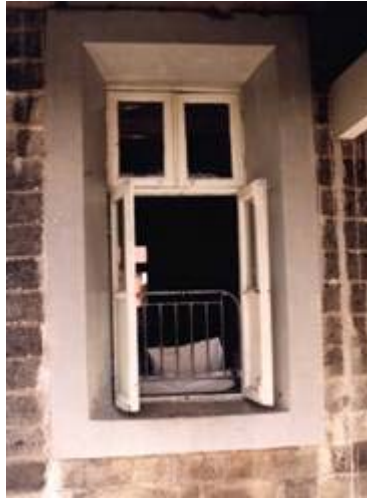
Fig. 13 The hospital window
